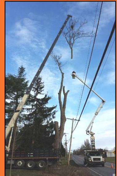
Tree removal needs to be performed by skilled professionals
