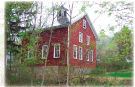
Mansfield Township is home to the Port Murray Historic District (above) and the Beattystown Historic District (below) which are both listed on the National and State Registers as examples of 18th and 19th century vernacular architecture.
