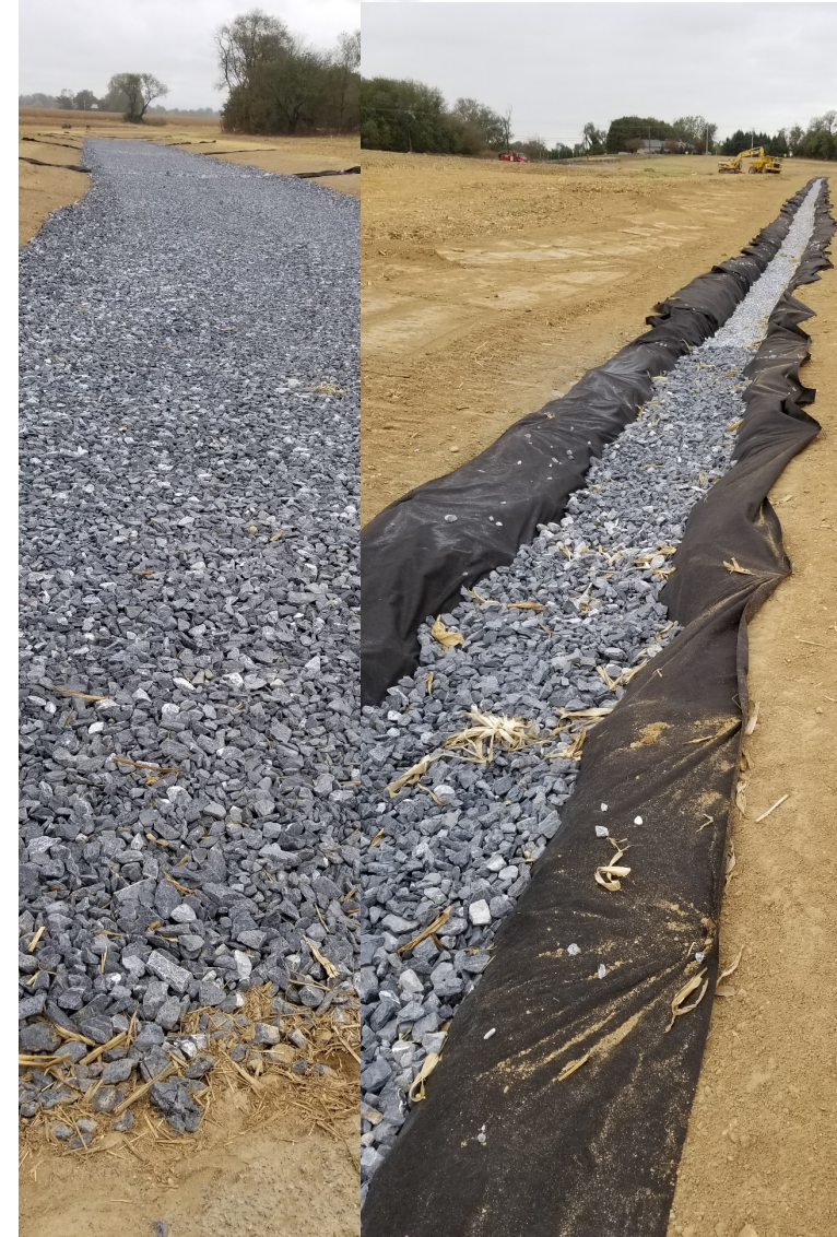
Example of geotextile separation
