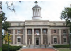
PLAINFIELD CITY HALL PLAINFIELD, NEW JERSEY
