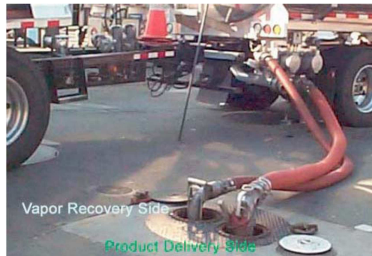
FIGURE 4: Two-Point Delivery (not coaxial)
