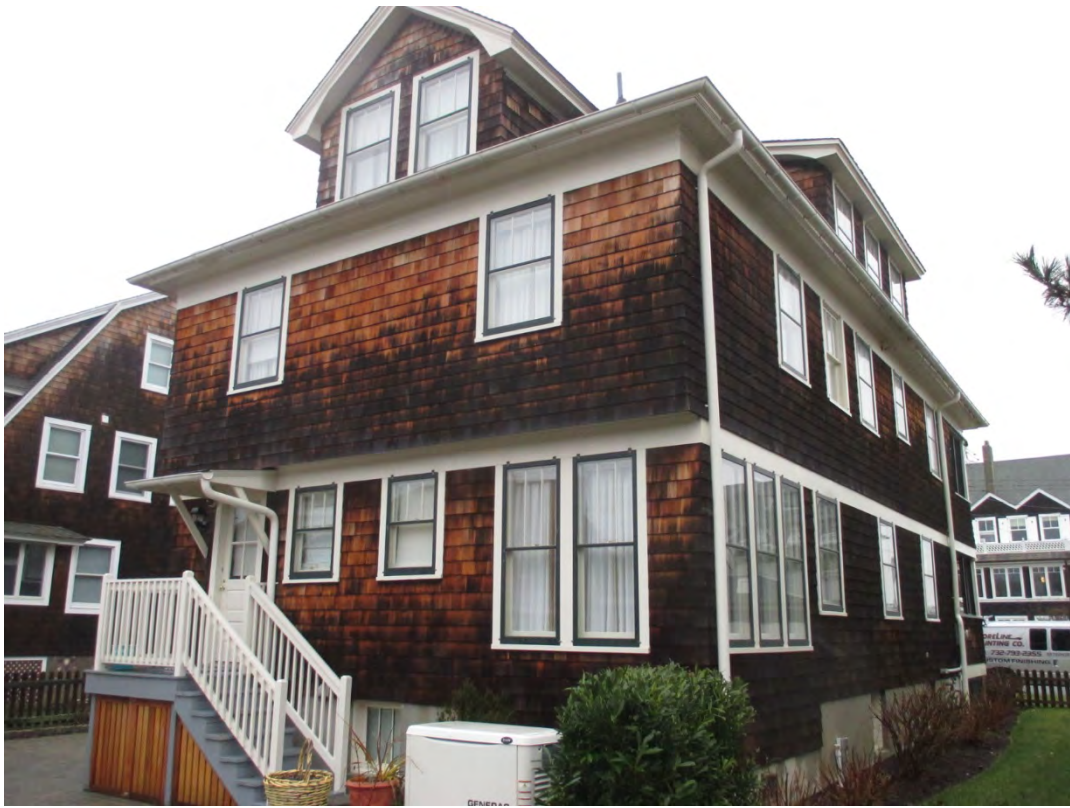
L. Ron Hubbard Residence, Borough of Bay Head, Ocean County Photo # 5
