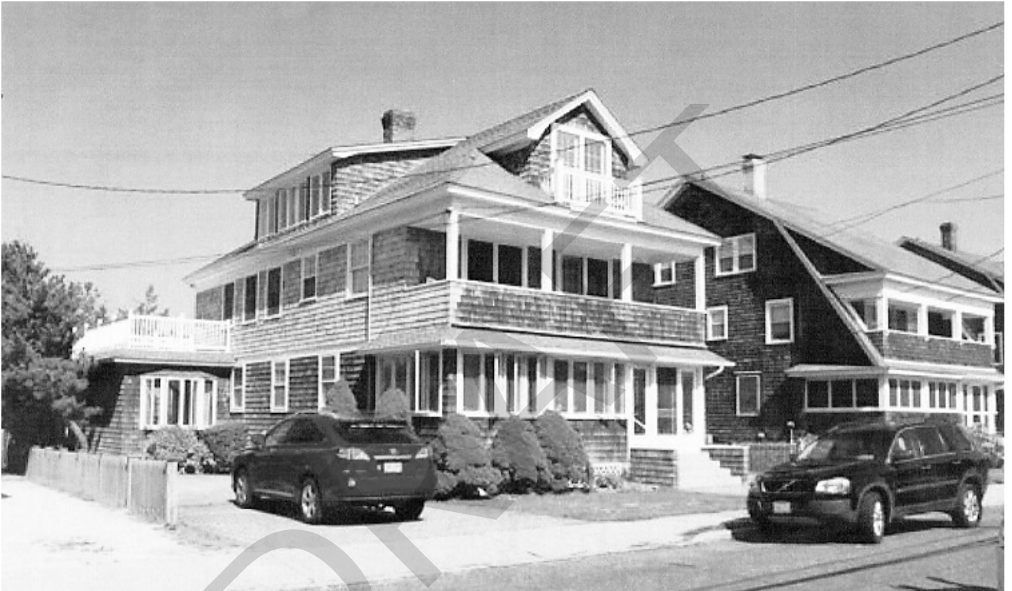
Historical Photograph 2. Front elevation of house prior to restoration (ca. 2010), showing enclosed porch, family room addition, and other alterations.
