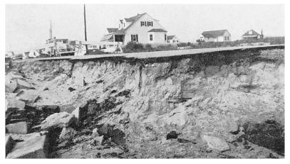
B. Wave erosion at Ocean City.
