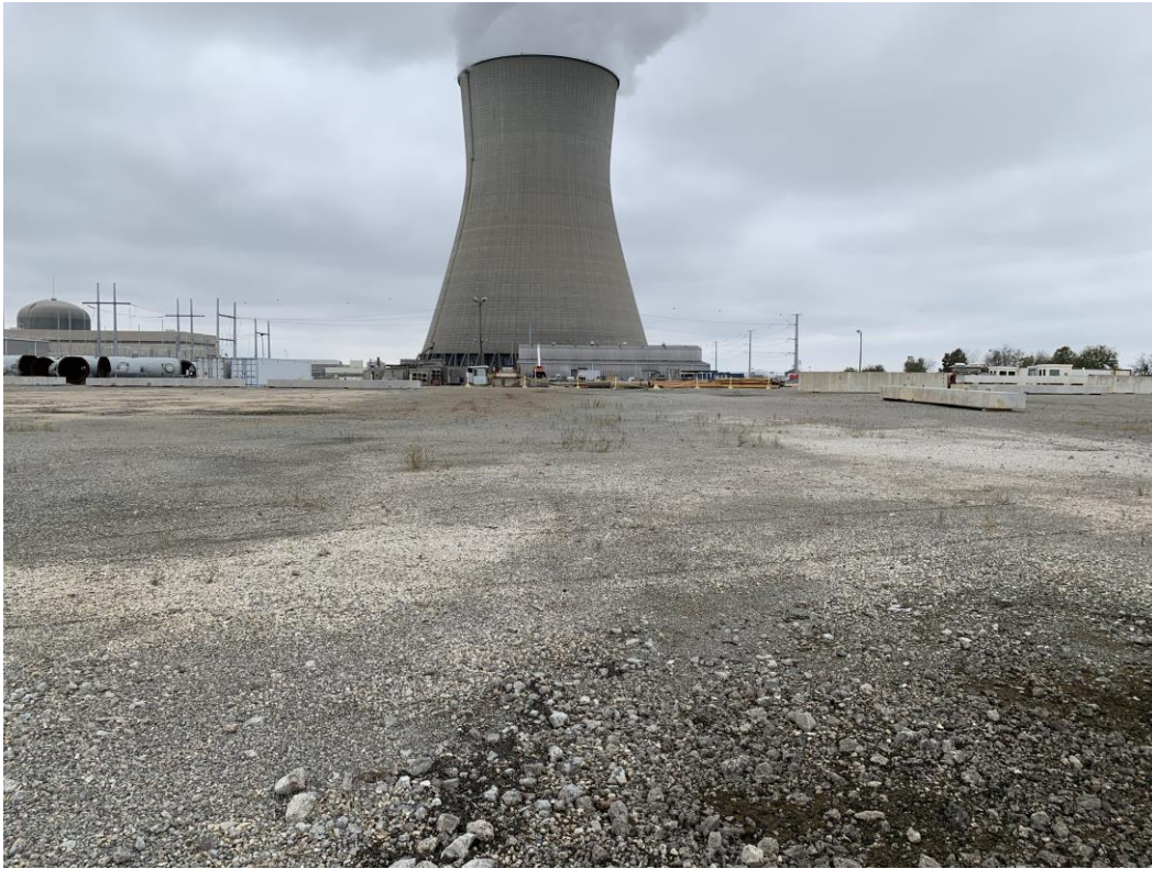
Photo looking west into the PSEG Nuclear laydown/emergency preparation area.
