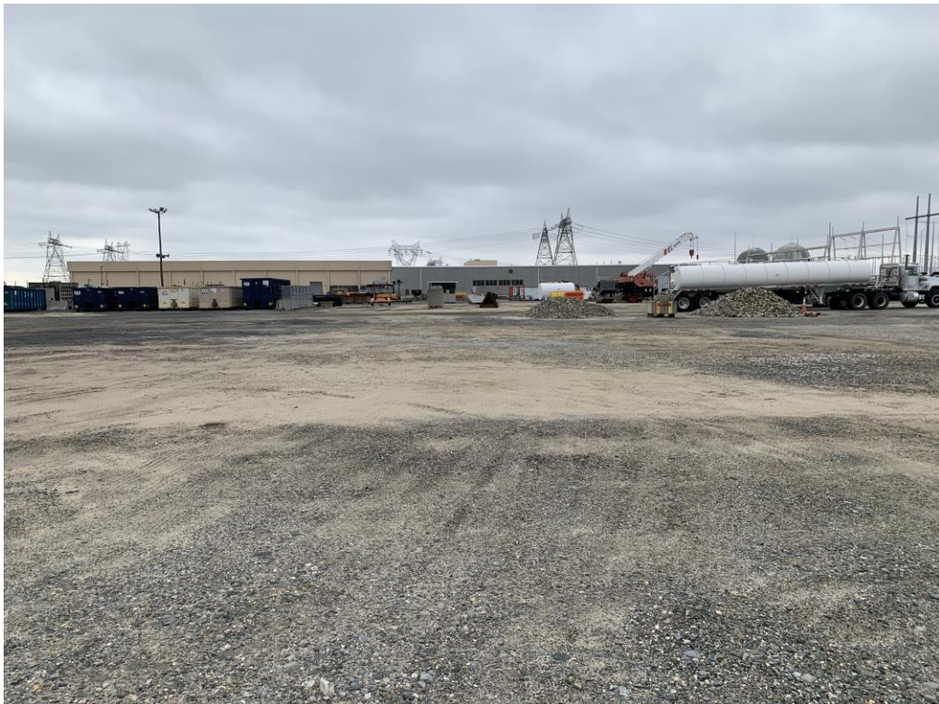
Photo looking south into a PSEG Nuclear laydown/emergency preparation area.
