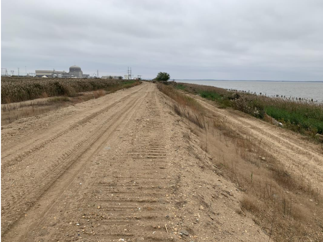
Photo taken looking south/southwest towards the access road below the USACE CDF Cell No.3 western berm. Note Delaware River and shoreline coastal wetlands on the right.
