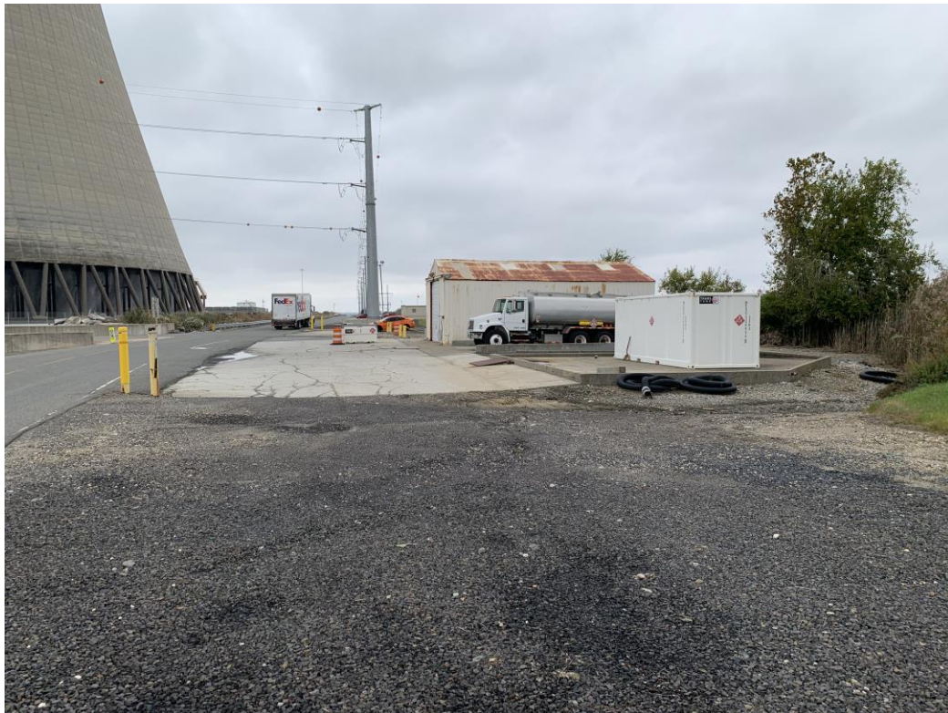
Photo looking west towards a PSEG Nuclear maintenance building.
