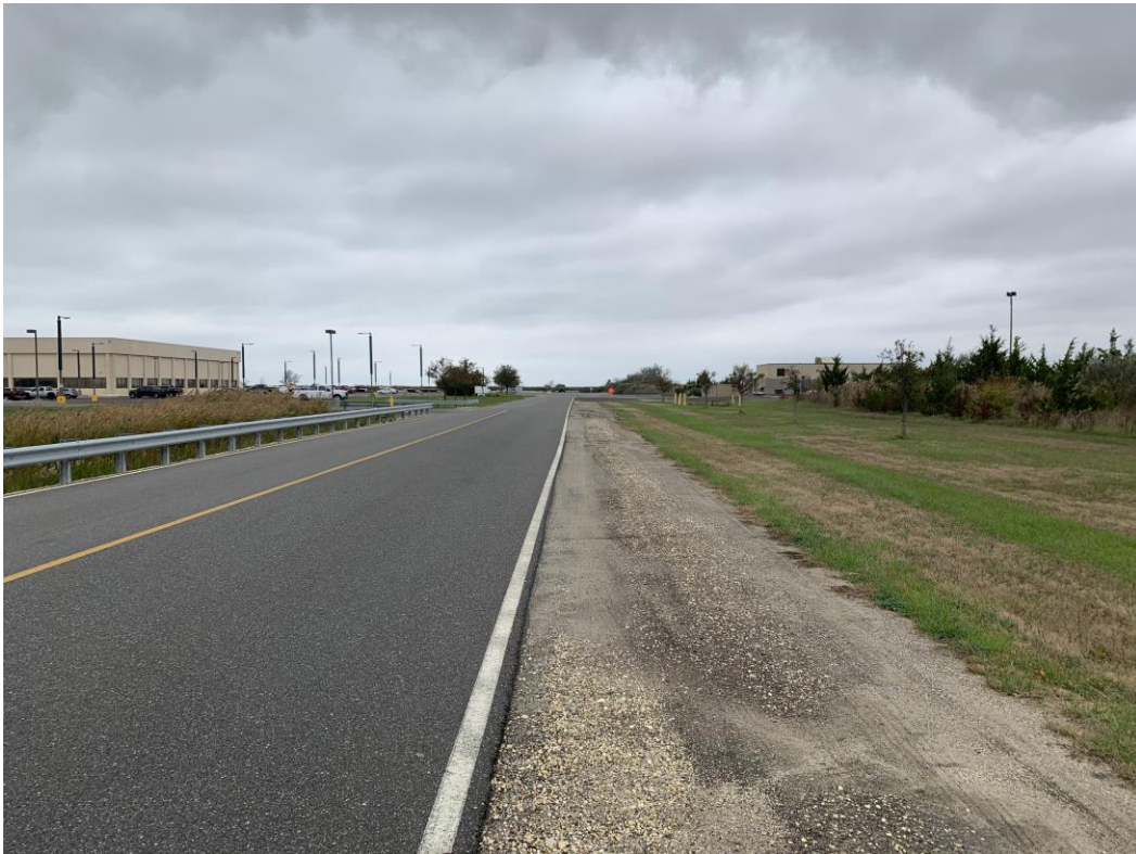
Photo looking north along PSEG Nuclear perimeter road.
