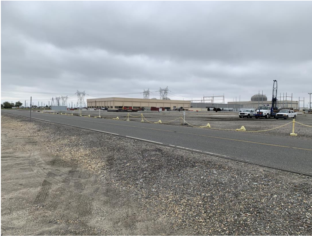
Photo looking southwest over the PSEG Nuclear laydown/emergency preparation area, towards the PSEG Nuclear admin building.
