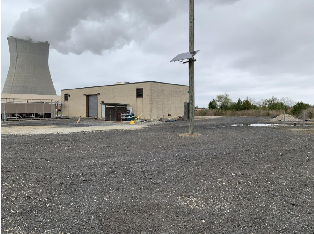
Photo looking northwest towards the PSEG Nuclear chill water building.
