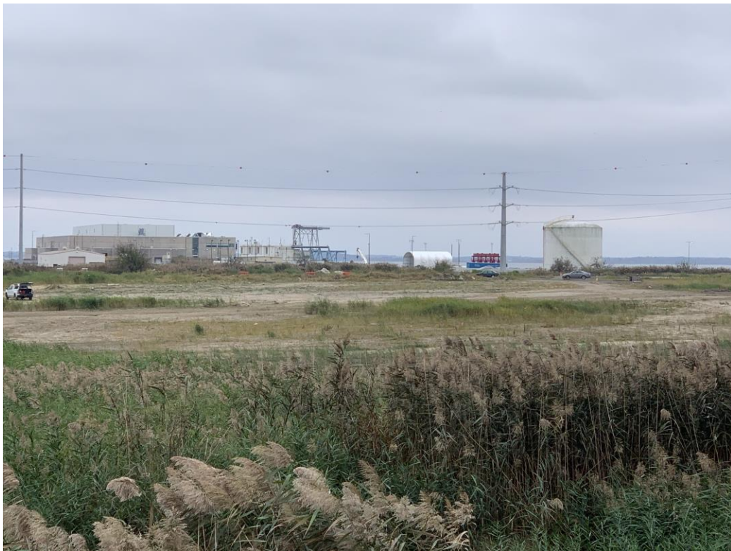
Photo looking south into the PSEG CDF. Photo taken from the top of the USACE CDF Cell No.3 southern berm.
