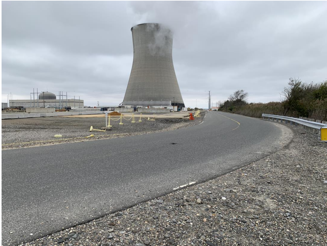
Photo looking west along the PSEG Nuclear perimeter road.
