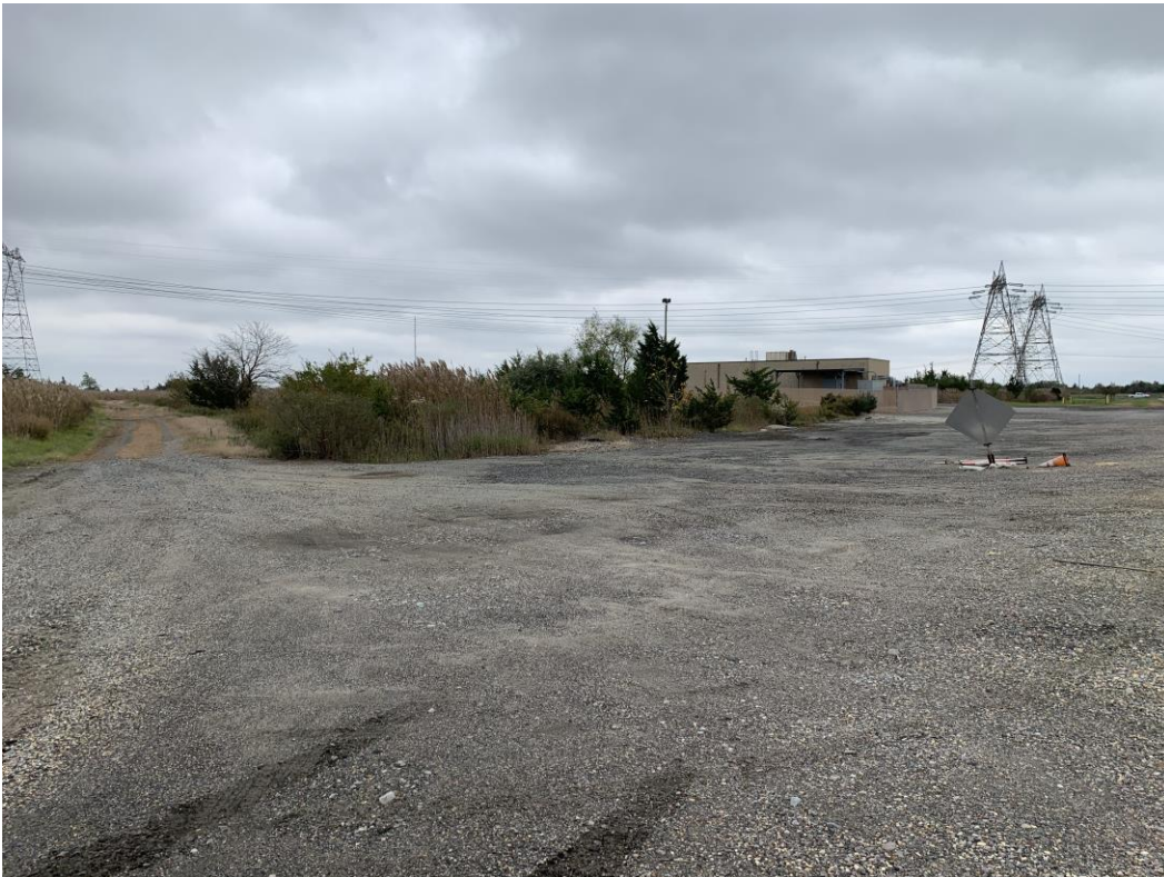
Photo looking southwest towards PSEG Nuclear chill water building. Note small roadside swale.
