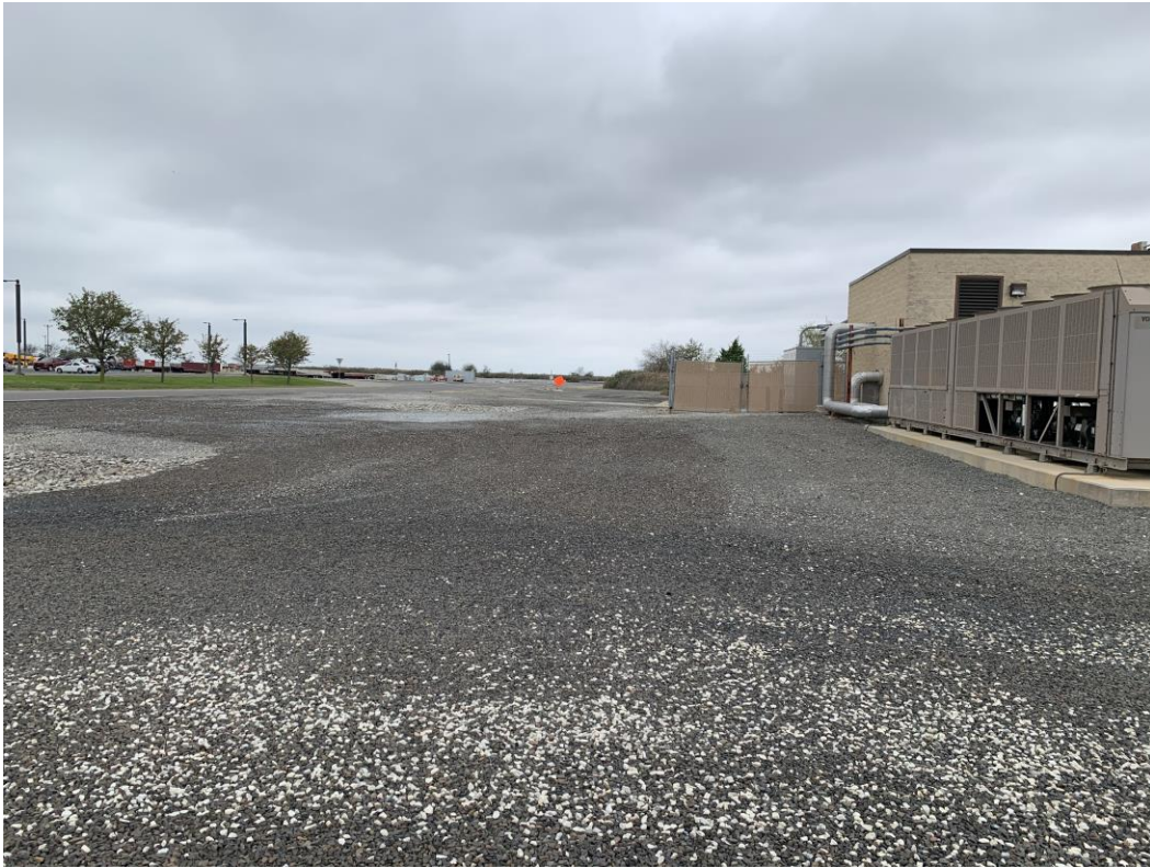
Photo looking north past the PSEG Nuclear chill water building.
