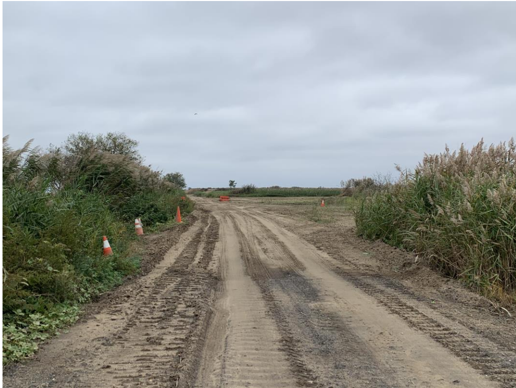
Photo looking north along the existing maintained access road to the PSEG and USACE CDF. Note coastal wetlands along Delaware River shoreline on the left.
