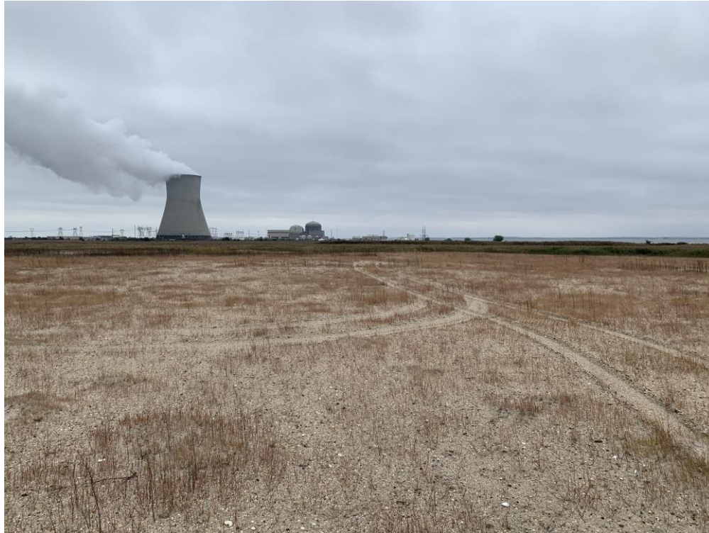
Photo looking south into the USACE CDF Cell No.3
