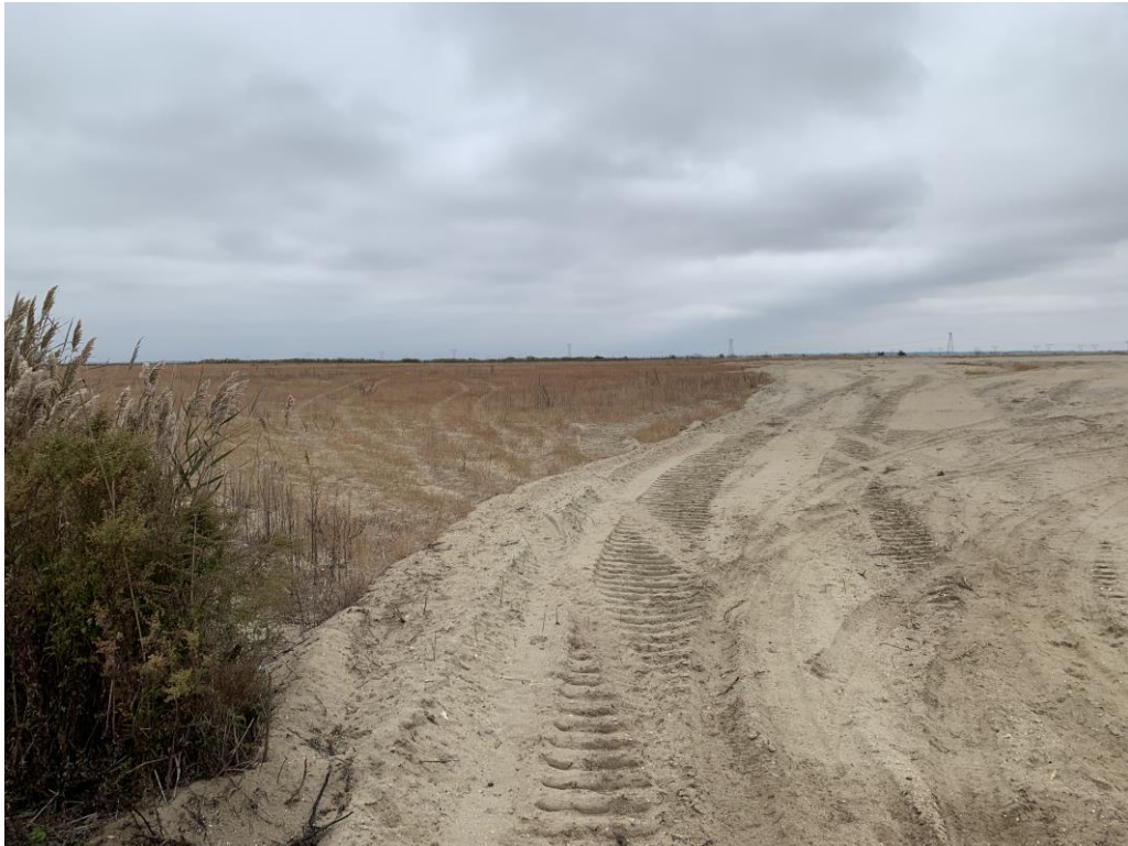
Photo looking northeast into the USACE CDF Cell No.3.
