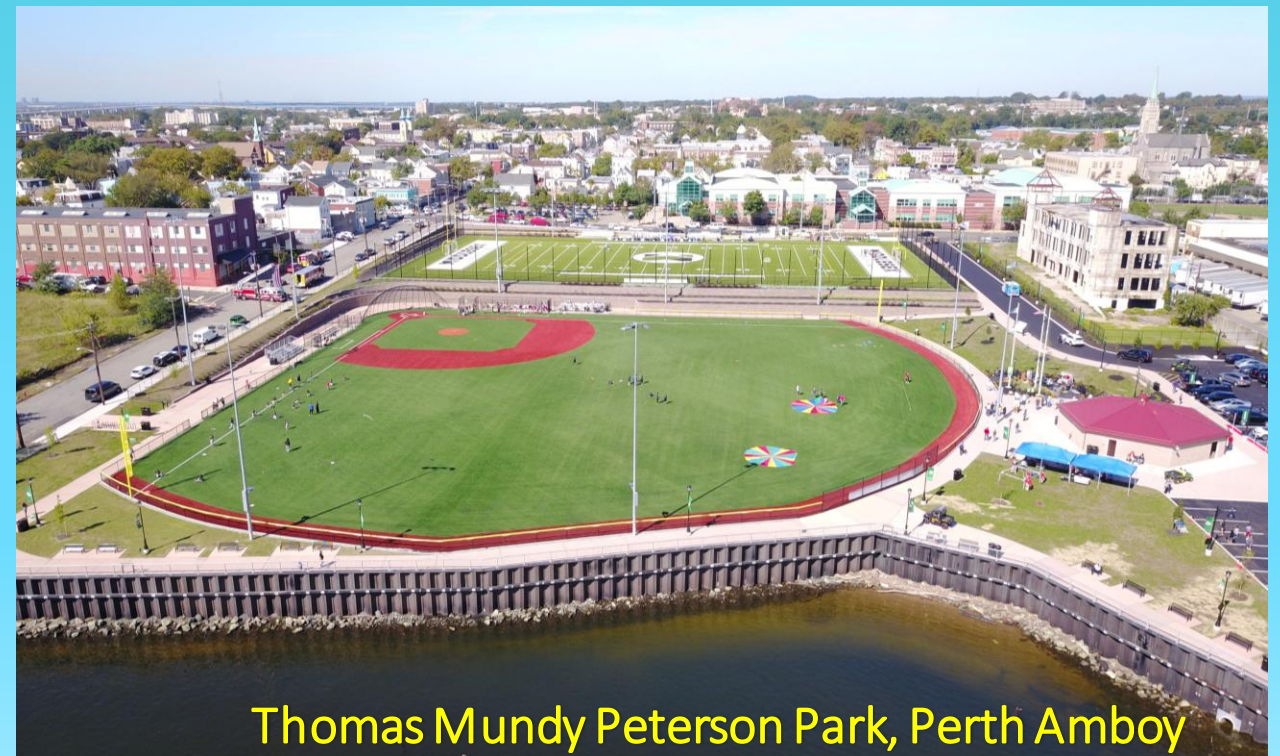
Former General Cable & Duane Marine Sites, Perth Amboy
