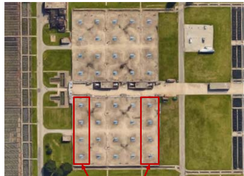
SWWPCP Aeration Train
