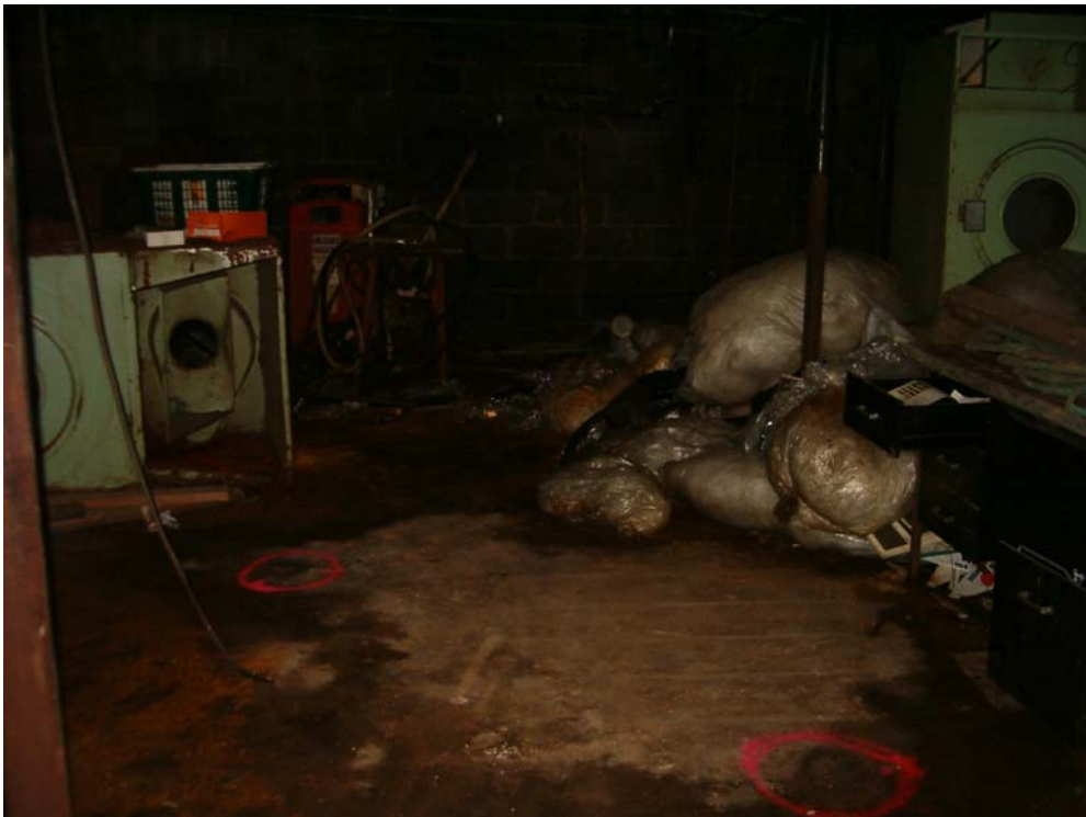
Photograph 5: Various debris in basement of former Topps Cleaners facility.
