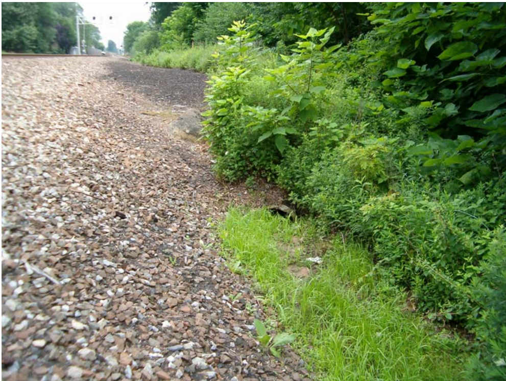
Photograph 3: Drainage swale along east side of New Jersey Transit property.
