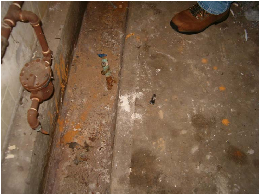
Photograph 4: Concrete floor trench within the former Topps Cleaners facility.
