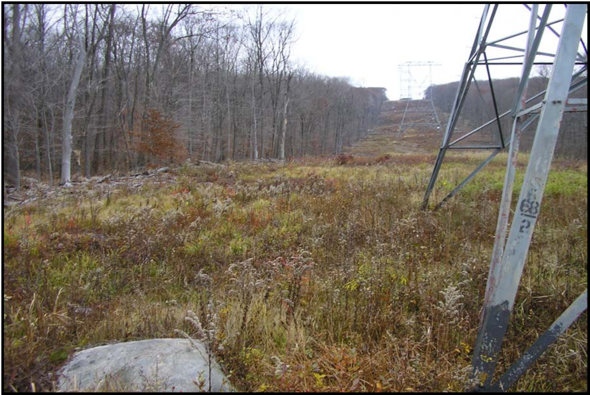
Photo of the Susquehanna - Roseland ROW in Rockaway Township.
