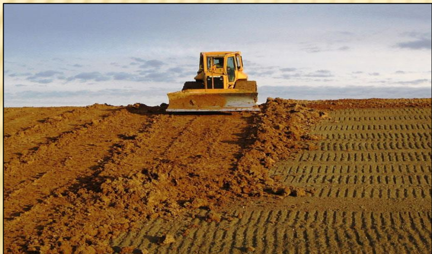
Permeable soil cover (Typ. 2' thick) is not an alternate means of addressing a public health or ecological risk – used where no such risk exists
