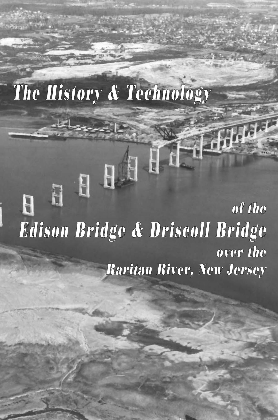
An aerial, black and white photograph showing the construction of a bridge over the Raritan River. Several large, rectangular concrete piers are visible in the water, with a crane on a barge positioned between them. The bridge deck is partially completed, extending from the right side of the frame towards the center. The surrounding landscape is a mix of urban development and open land.
