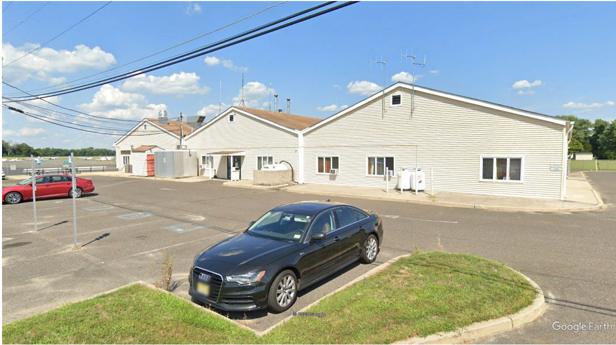
Office Building at South Jersey Regional Airport.
