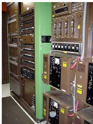
The replacement network will utilize Nortel DMS 100 Switches.
