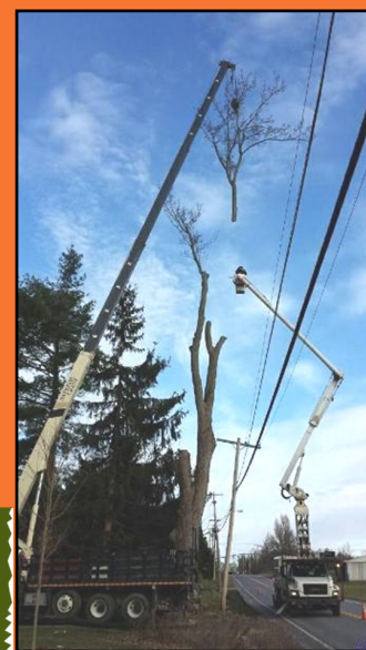
Employees must be line clearance certified to work near powerlines.
