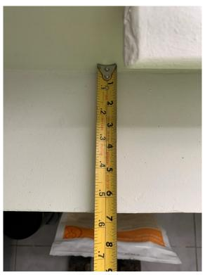
Photo 12. Protrusion of CMU Foundations Walls into Building (Typical Around Perimeter)
