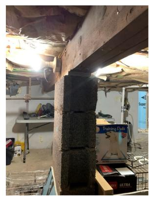
Photo 7. Girder with CMU Pedestal in East Crawl Space (Looking West)
