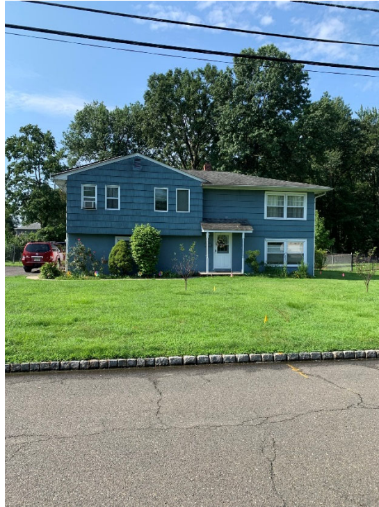
Photo 1. 10 Sylvan Road (Front of Building)
