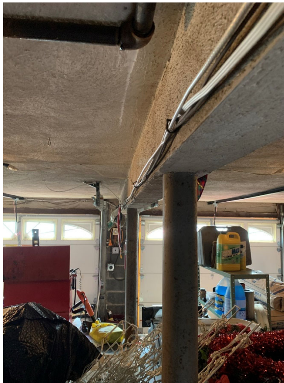
Photo 4. Garage Girder & Steel Post Columns (Looking East)
