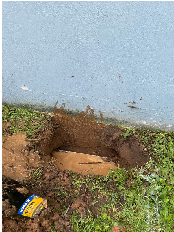
Photo 16. Test Pit TP-1 Conditions
