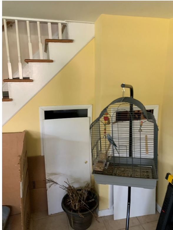
Photo 9. Boiler Room Beneath Stairs to Second Floor (Looking Southeast)
