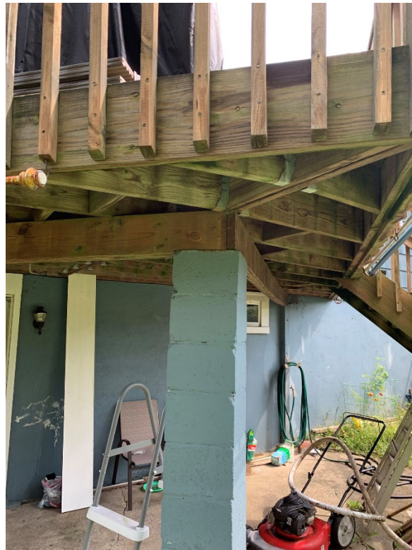
Photo 14. Rear Timber Deck Frame & Columns
