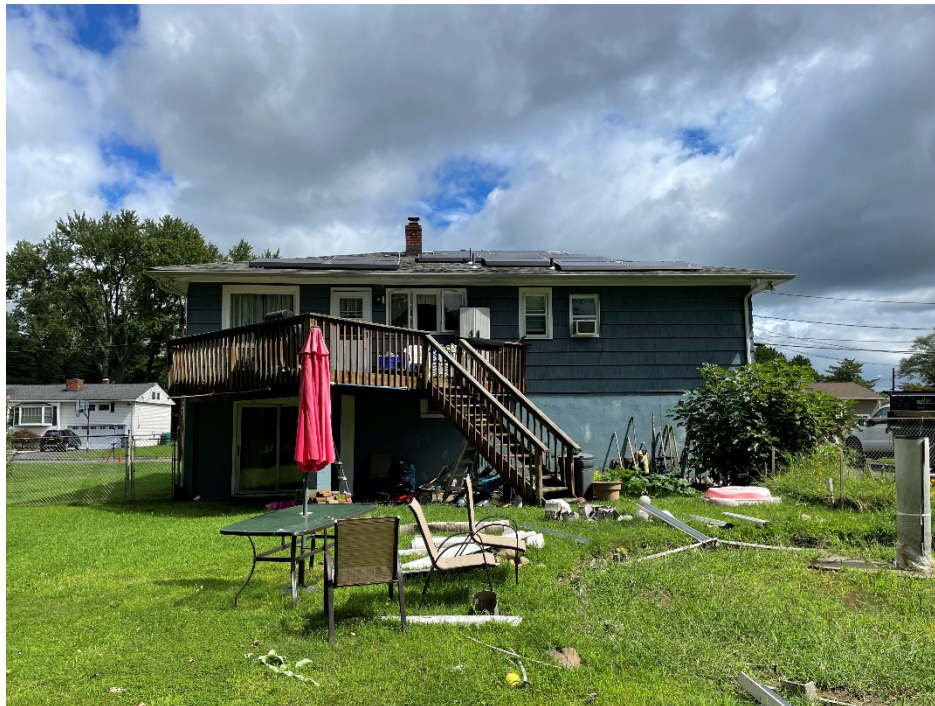
Photo 2. 10 Sylvan Road (Rear of Building)
