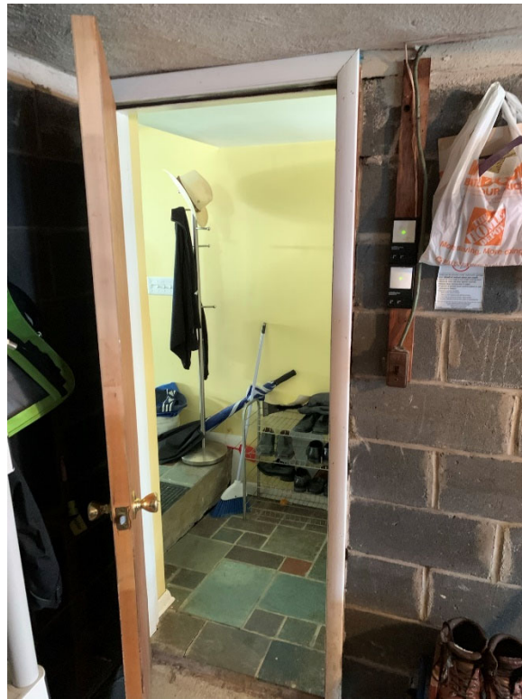
Photo 3. Garage Entrance Door & CMU Foundation Walls (Looking North)
