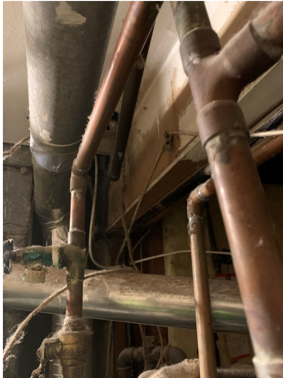
Photo 11. Timber Girder Above Boiler Room (Looking Northwest)
