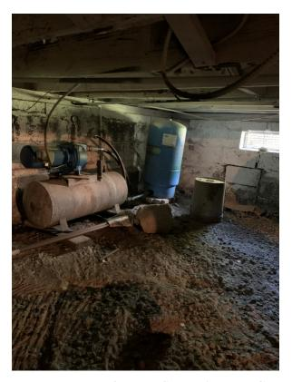
Photo 5. Water Well Pressure Tank & Pump System in Front Crawl (Looking North)
