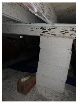
Photo 6. Timber Floor Joists & Girder on CMU Pedestal (Front Crawl Space)
