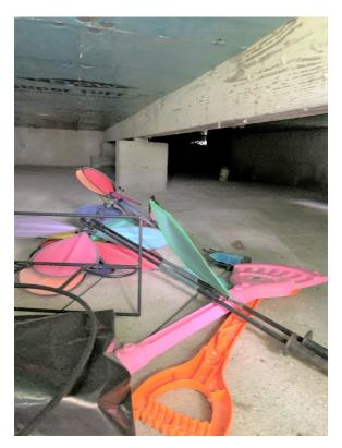
Photo 11. Timber Girder & CMU Pedestals in Rear Crawl Space (Looking Northeast)
