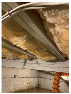
Photo 6. Typical Subfloor Above Front Crawl Space 22
