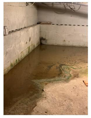
Photo 7. Standing Water in Northeast Corner of Front Crawl Space (Looking East)
