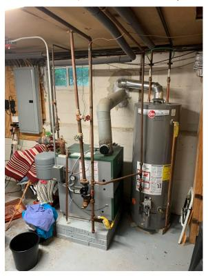
Photo 6. Basement Foundation Wall with Boiler, Hot Water Heater & Elec. Panel (Looking West)
