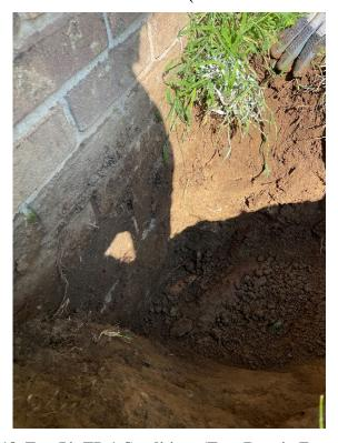
**Photo 18. Test Pit TP-1 Conditions (Tree Root in Excavation)**
