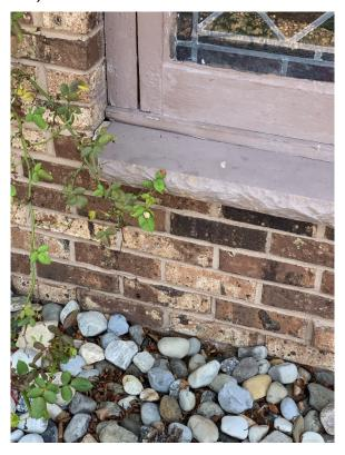
Photo 14. Crack in Brick Façade Below Window on West Wall of Rear Addition (Looking East)
