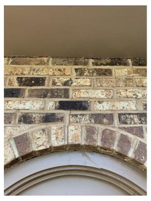
Photo 13. Crack in Brick Façade Above Window on West Wall of Rear Addition (Looking East)
