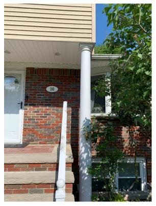
Photo 4. Column Supporting Second Floor Overhang in Front of Building (Looking West)
