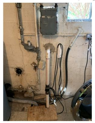
Photo 8. CMU Foundation Walls in Basement with Gas Meter & Sump Pit (Looking East)
