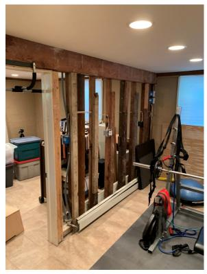
Photo 6. Unfinished Partition Wall in Basement with Girder & Steel Post (Looking Southeast)
