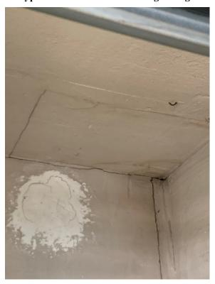
Photo 12. Cracks & Water Staining on South Wall of Garage (Southeast Corner)
