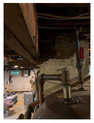
Photo 7. (2) 2x8 Timber Girder in Basement
