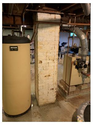
Photo 9. Water Heater (Left) and Boiler (Right) in Basement
