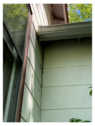
Photo 13. Separation of East Addition from Main Building Frame
