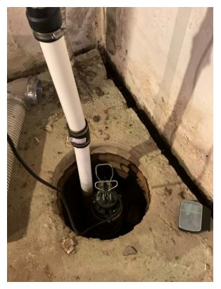
Photo 5. Sump Pump in Basement (Southwest Corner)
