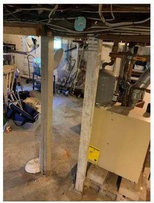
Photo 8. Timber 4x4 Girder Support Posts (Typ.)
