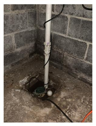
Photo 7. Sump Pump in Crawl Space (Northwest Corner)
