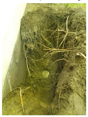
**Photo 15. Test Pit TP-2 Foundation Conditions**
