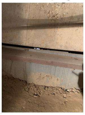
Photo 10. Shoring Below Concrete Beam (West Edge of Crawl Space)
