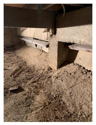
Photo 9. Concrete Beam and Column (West Edge of Crawl Space)
