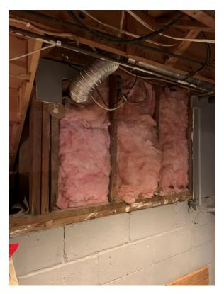
Photo 7. Lowered CMU Foundation Wall in Basement (Looking South)
