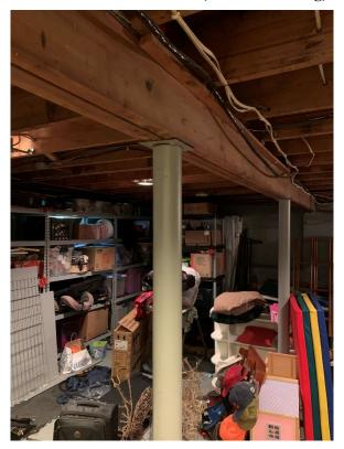
Photo 4. Basement Girders, Columns & Subfloor (Looking Northwest)
