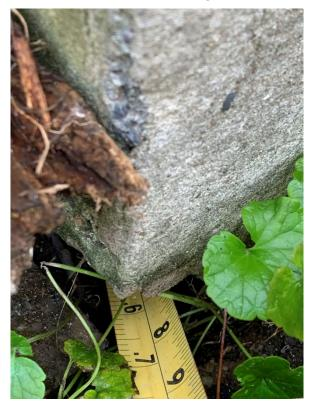
Photo 10. Hole in Basement Foundation Wall (Northwest Corner)
