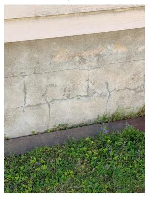
Photo 10. Stucco Cracks in West Exterior Wall
