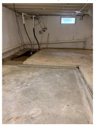
**Photo 4. Basement Concrete Floors with Differing Elevations**
