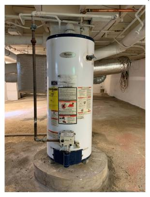
Photo 6. Water Heater on Concrete Platform (Center of Basement)
