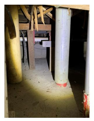
Photo 9. Additional Timber Beam in Central Crawl Space (Looking South)
