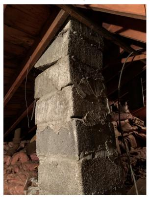
Photo 14. Damaged Exhaust Chimney Extending Through Attic (Looking Northwest)
