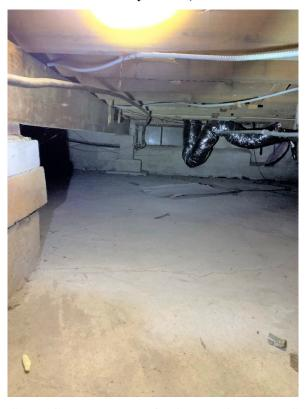
Photo 8. Central Crawl Space Concrete Walls & Timber First-Floor Subfloor (Looking West)
