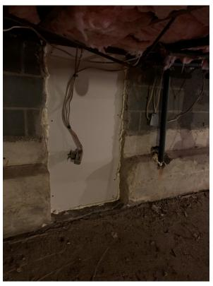
Photo 14. Boarded Up Opening in Crawl Space South Wall 26
