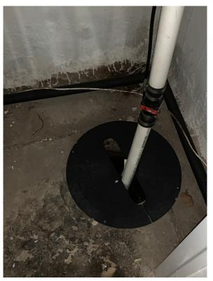
Photo 6. Sump Pump in Unfinished Portion of Basement (Typ.) 22
