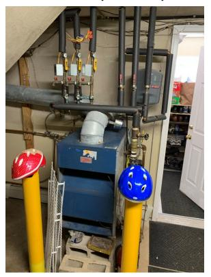
Photo 10. Boiler in Garage (Rear Wall)
