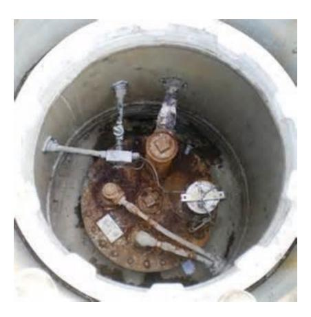
Check valve at the dispenser and top of the tank – product remains in line when not in use
