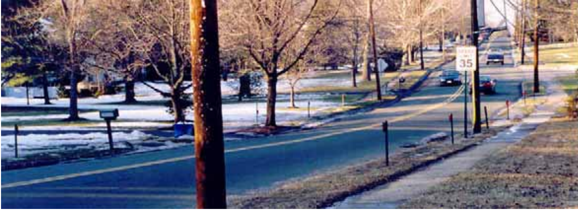
Figure 5. Roadside reflectors intended to deter deer from roads at night.
