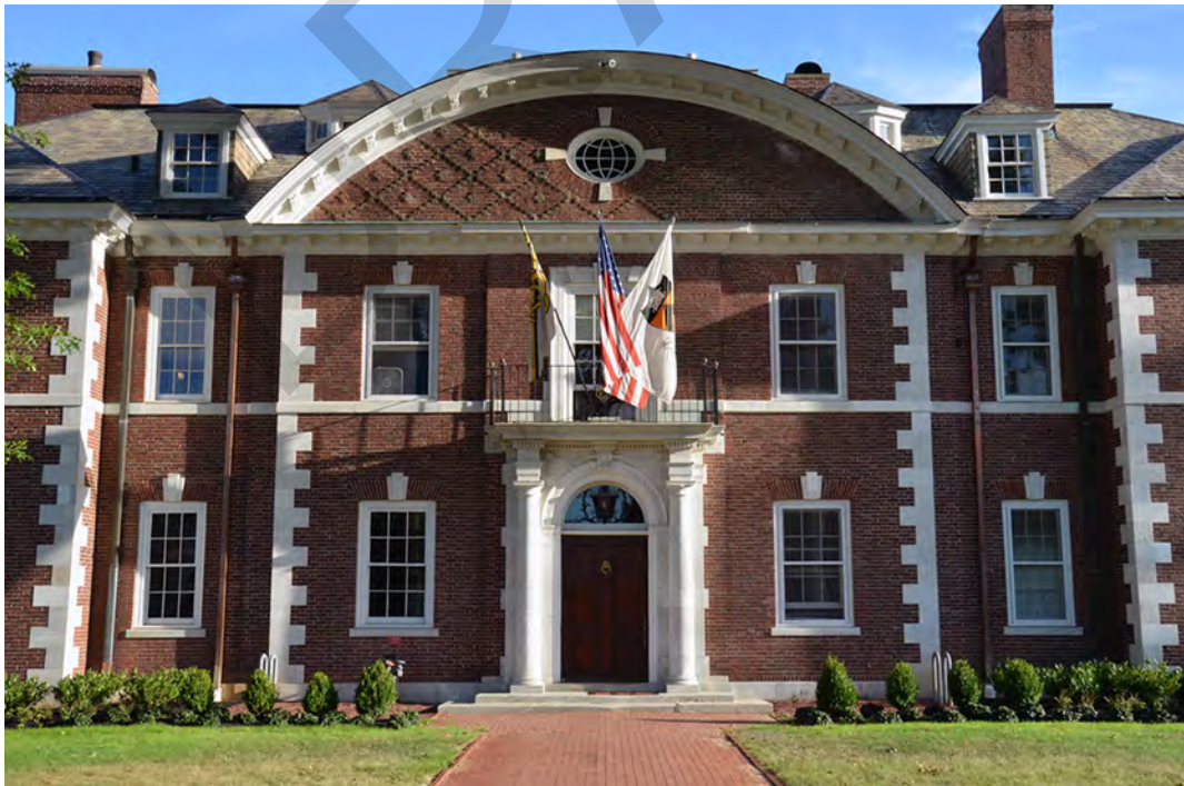
4.2 Cottage Facade S CW Zink 2016
