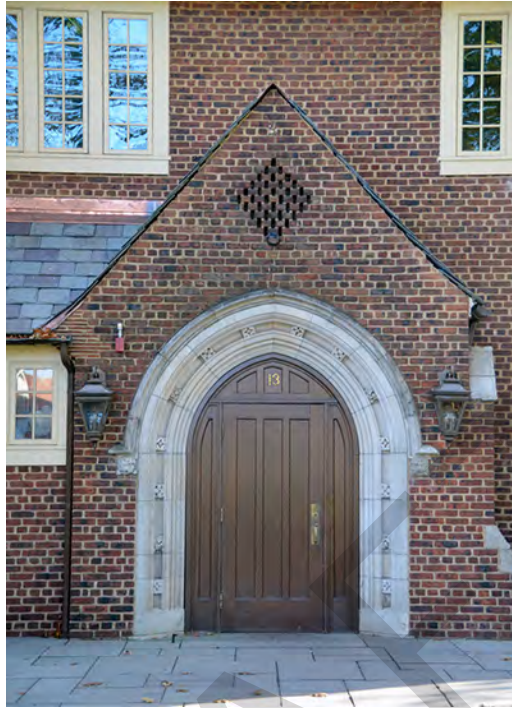
11.2 Tower Club Entrance S CW Zink 2016
