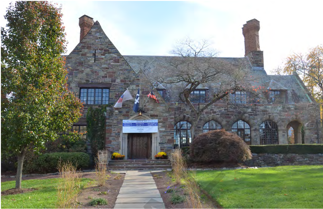
14.1 Cloister Inn Facade S CW Zink 2016
