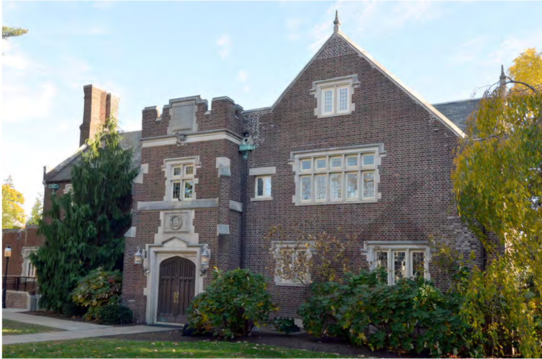
7.2 Campus Club Facade SE CW Zink 2016
