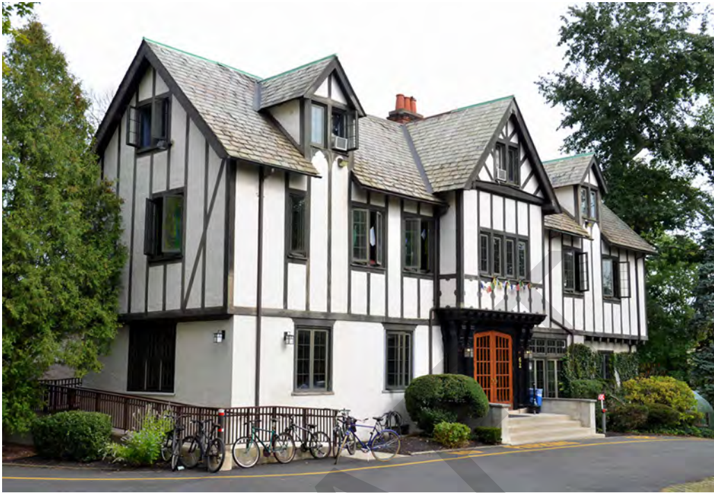
13.1 Terrace Club Facade SE CW Zink 2016
