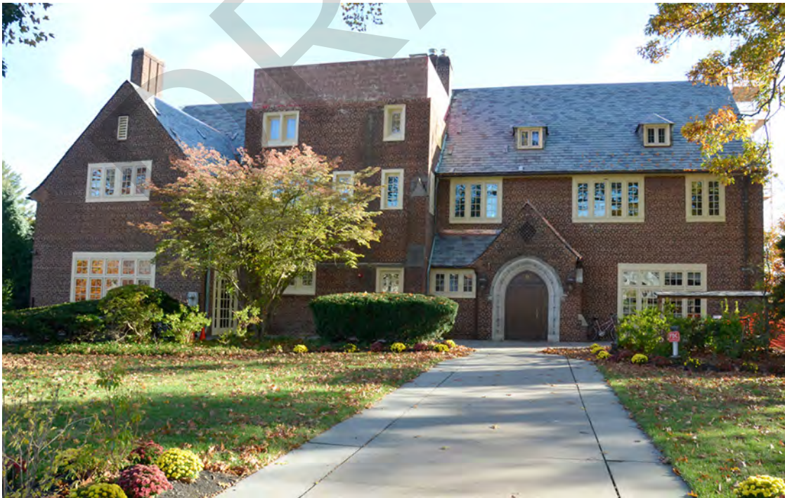
11.1 Tower Club Facade S CW Zink 2016
