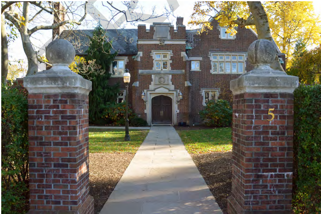
7.1 Campus Club Facade S CW Zink 2016
