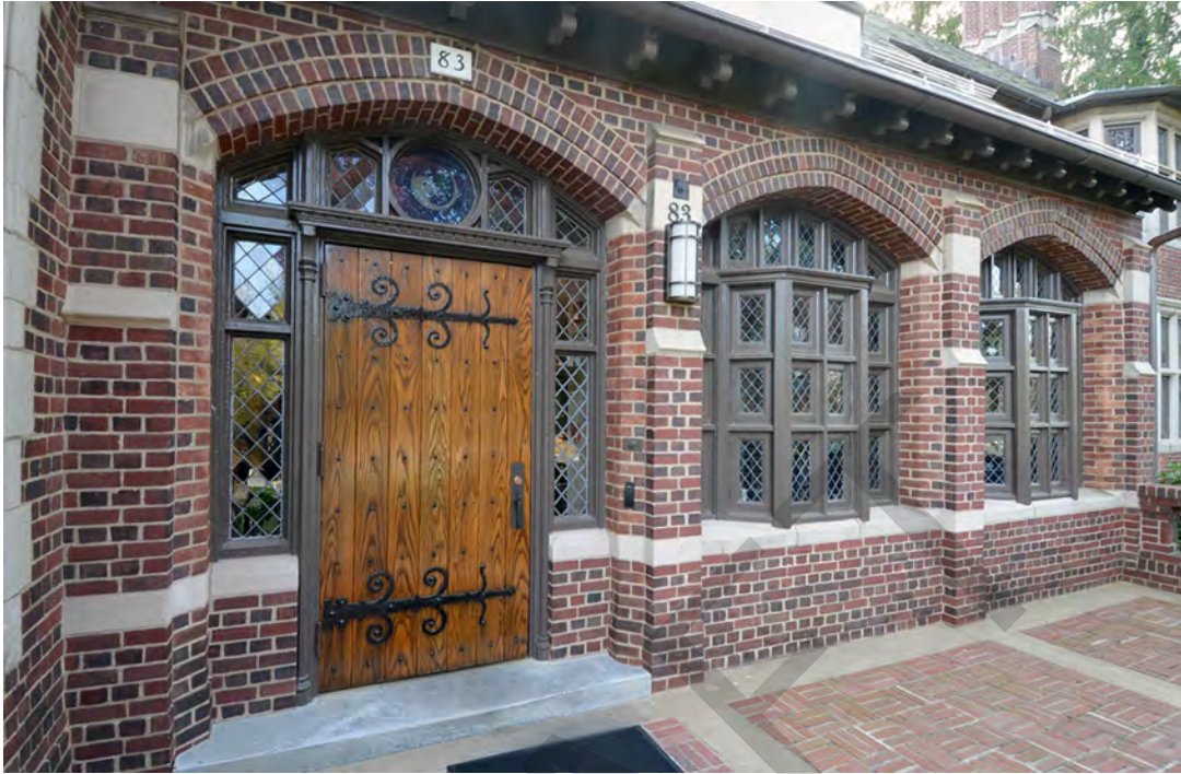
15.4 Key & Seal Clubhouse Entrance SW CW Zink 2016
