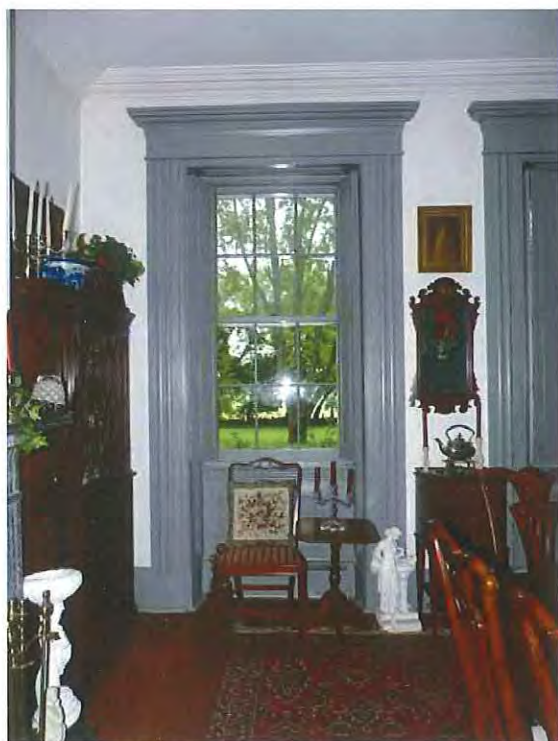
NJ_BURLINGTON_RIDGWAY, HOUSE, WILLIAM_0025 Detail facing north in the northwest parlor showing the typical parlor window trim and decorative cornice.
