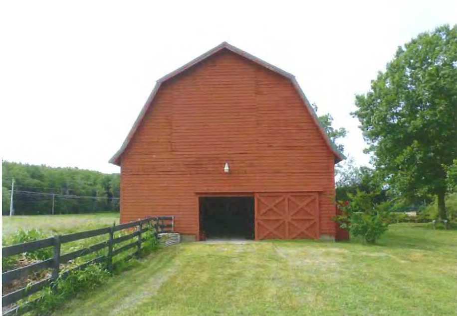
NJ_BURLINGTON_RIDGWAY, HOUSE, WILLIAM_0048 View facing south showing the north elevation of the barn.
