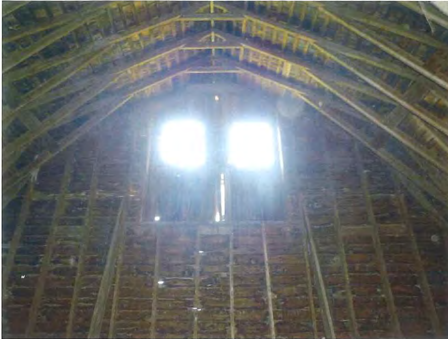
NJ_BURLINGTON_RIDGWAY, HOUSE, WILLIAM_0052 View facing south in the second floor of the barn.
