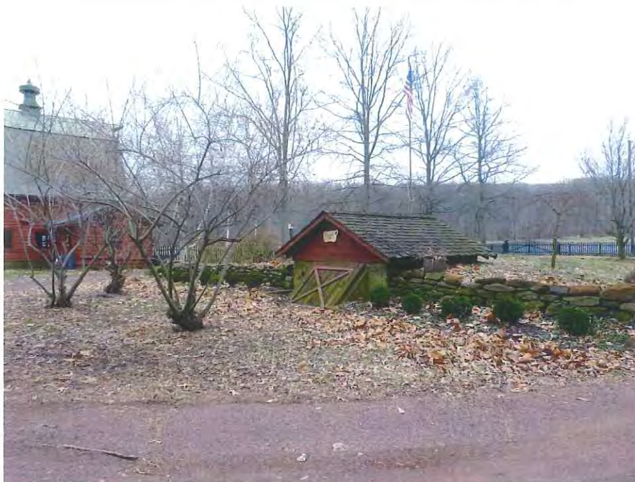
NJ_BURLINGTON-RIDGWAY, HOUSE, WILLIAM_0010 View facing southeast showing the pump house and the barn at left.
