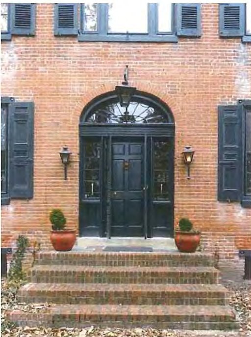
NJ_BURLINGTON-RIDGWAY, HOUSE, WILLIAM_0013 Detail facing north showing the main entrance on the south elevation.
