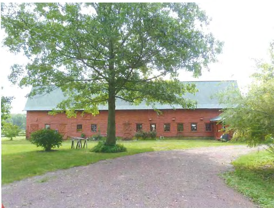
NJ_BURLINGTON_RIDGWAY, HOUSE, WILLIAM_0047 View facing east showing the west elevation of the barn.
