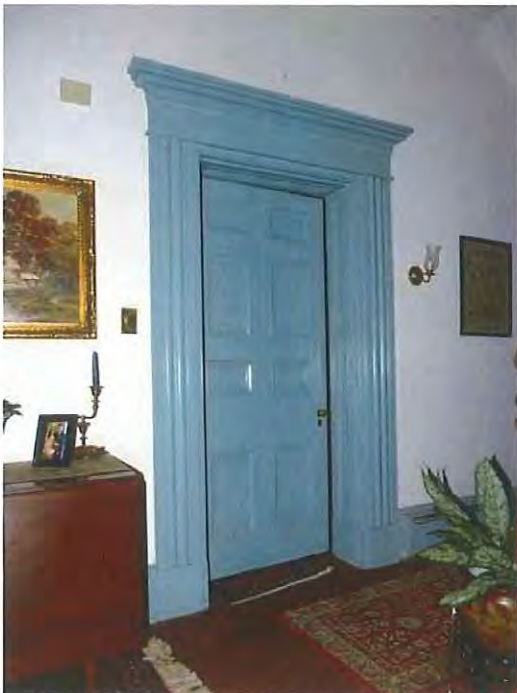
NJ_BURLINGTON-RIDGWAY, HOUSE, WILLIAM_0021 View facing southeast in the front entrance hall on the first floor showing an eight-panel door and trim.
