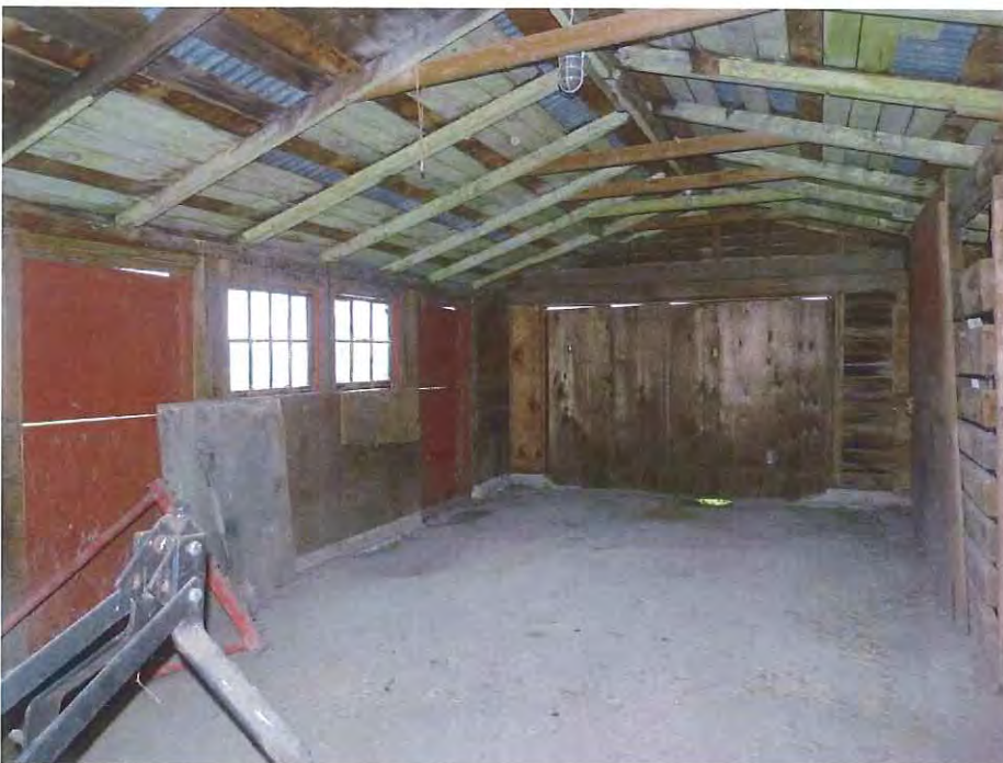
NJ_BURLINGTON_RIDGWAY, HOUSE, WILLIAM_0055 View facing west in the shed.
