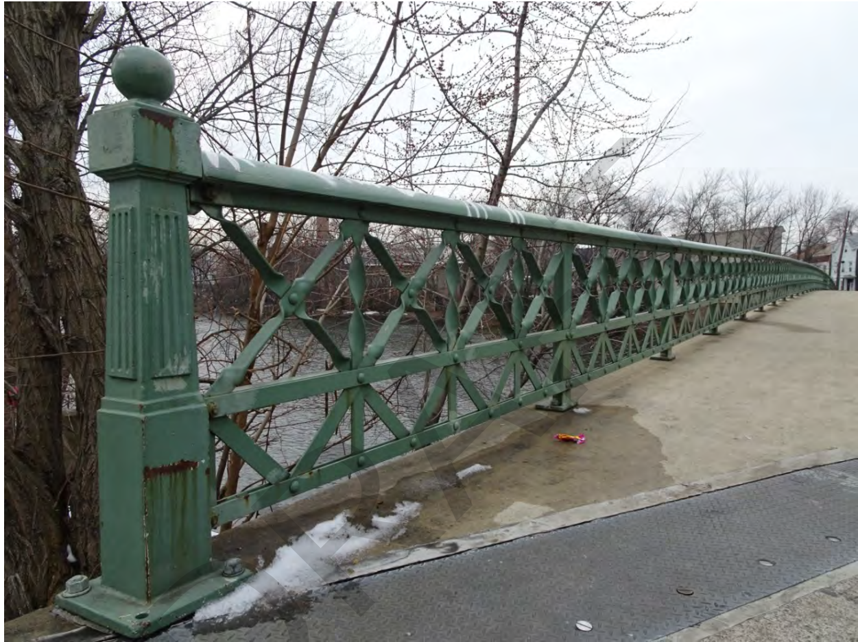
Photograph 11. View of original newel post and pedestrian railing, looking west across the Passaic River.
