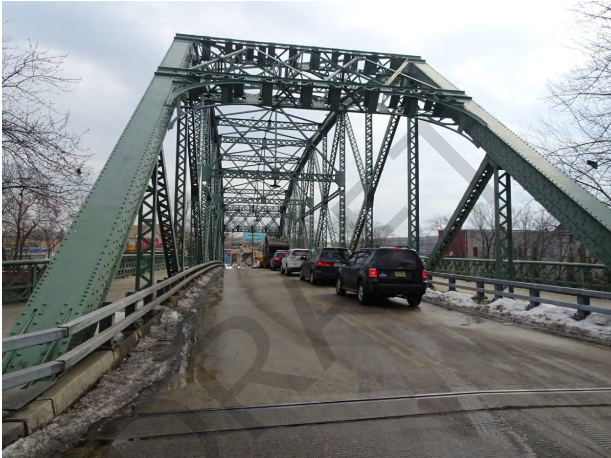
Photograph 5. View of bridge and deck from North Straight Street, looking southeast.
