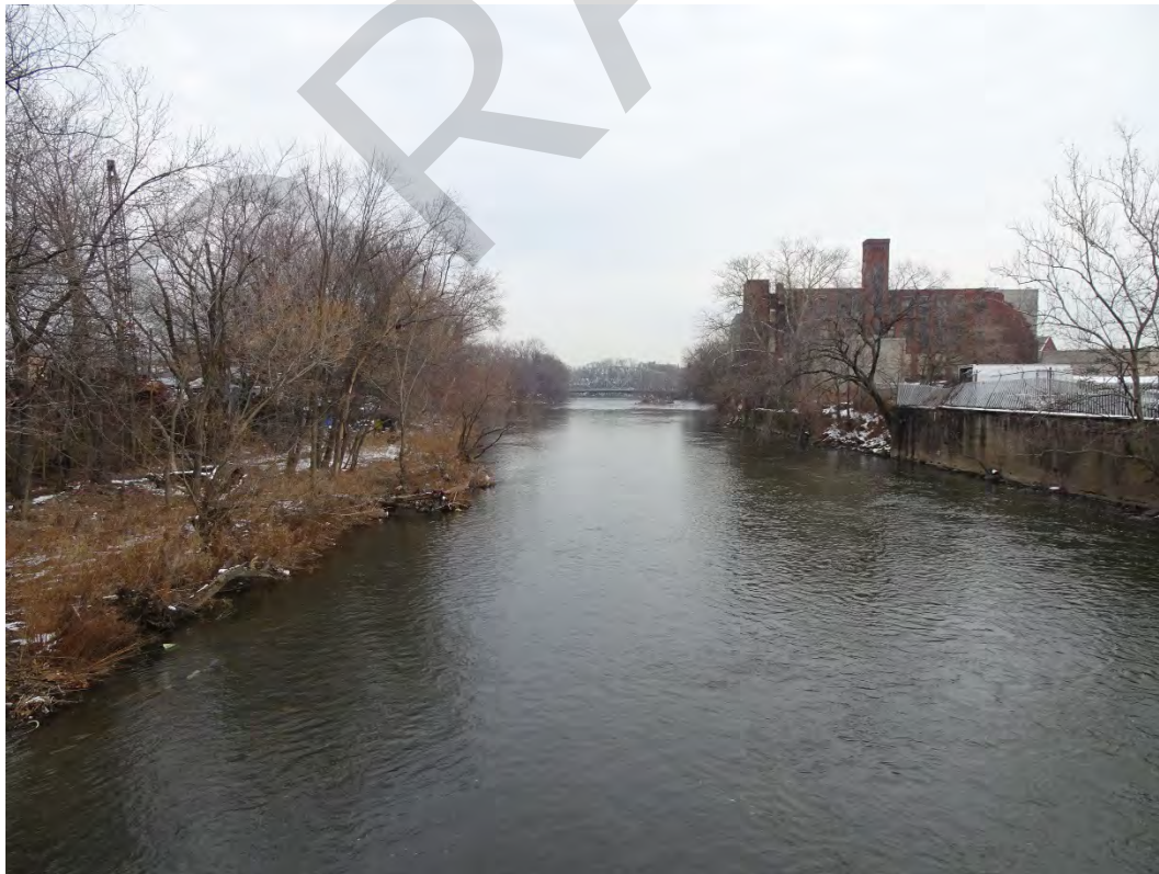
Straight Street Bridge over the Passaic River, City of Paterson, Passaic County Photo #15
