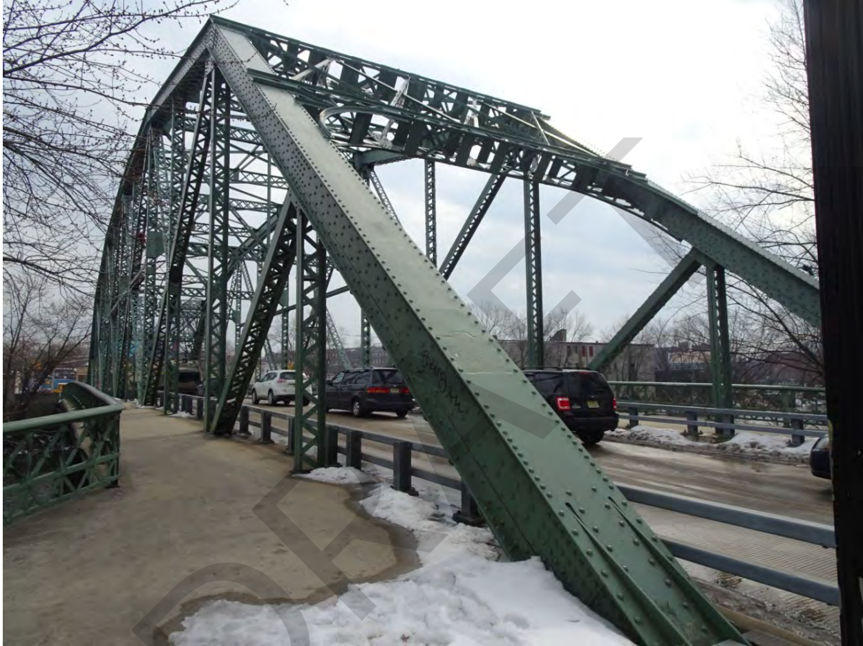
Photograph 3. View of bridge and northeast sidewalk from North Bridge Street, looking southeast.
