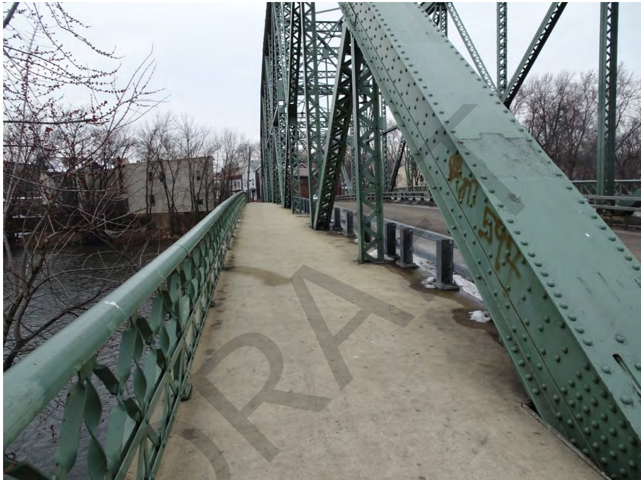
Photograph 10. View of the southeast pedestrian sidewalk, looking northwest.
