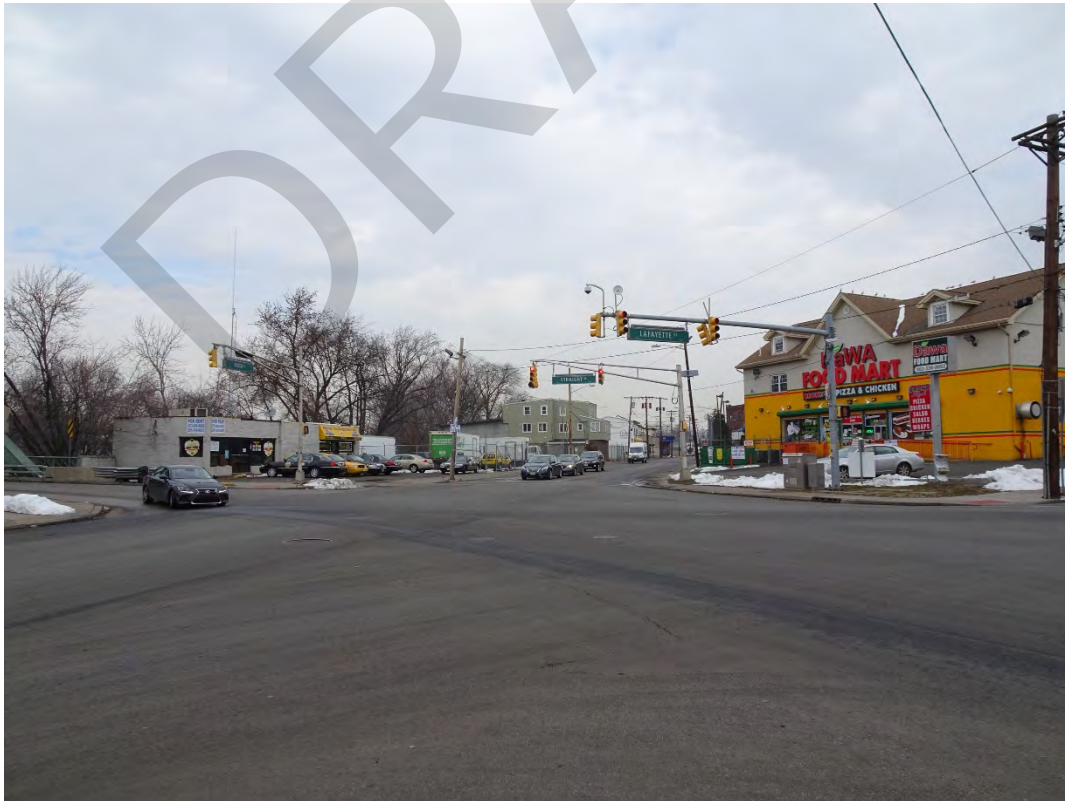
Straight Street Bridge over the Passaic River, City of Paterson, Passaic County Photo #4
