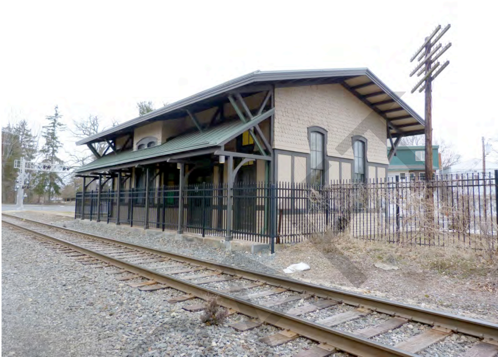
Photograph 0005: View of the west and south elevations and railroad tracks, camera facing northeast.
