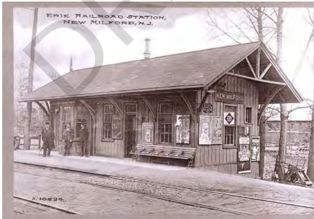
Supplemental Photograph 13: New Milford Depot (c.1880), Erie Railroad. Note the variation on the form, with the projecting bay offset to the left, as well as the overhanging eaves, brackets, and board-and-batten siding.
