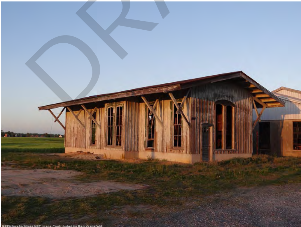
Supplemental Photograph 8: Woodstown Depot (c.1885, moved), Woodstown and Swedesboro Railroad. Note the form, projecting bay, extended eaves, knee braces, board-and-batten siding similar to Glassboro. Not shown is a garage entrance on the opposite gable end that may have been a larger freight door.
