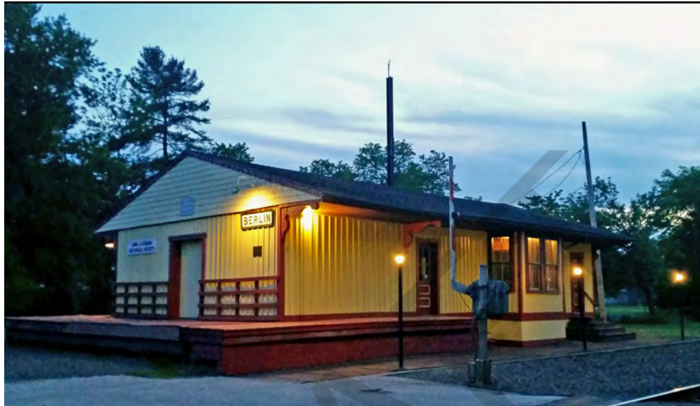
Supplemental Photograph 5: Long-A-Coming Depot (1856), Atlantic and Camden Rail Road Company. Note the board-and-batten siding, extended eaves, brackets, and projecting bay.
