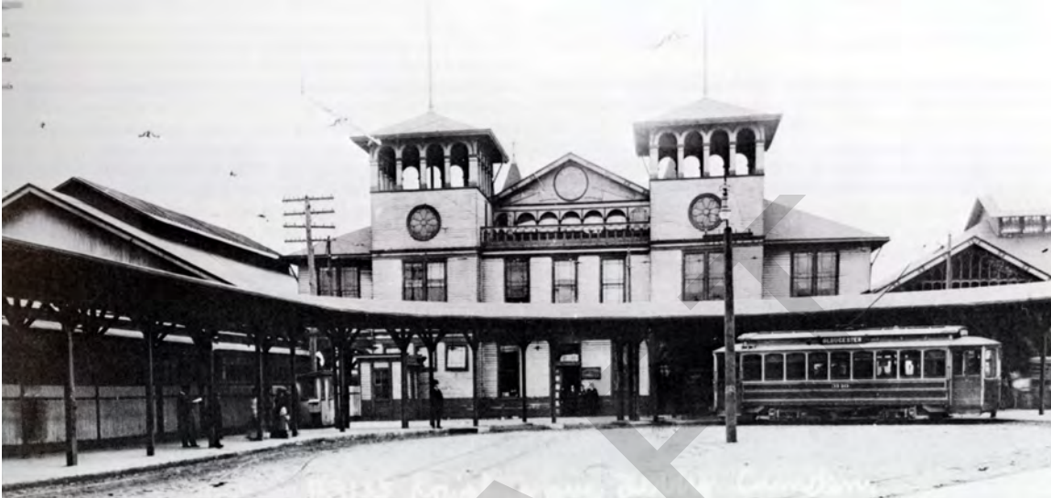
Supplemental Photograph 3: Camden Train Station, Camden, NJ. Demolished.
