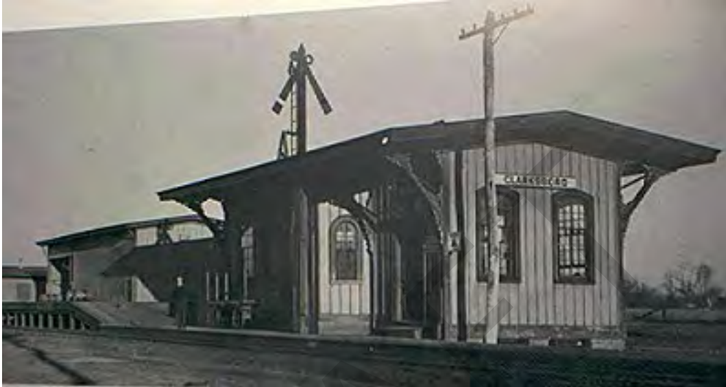
Supplemental Photograph 7: Clarksboro Depot (c.1869, demolished), WJRR. Note the center bay, projecting eaves and brackets, and the board-and-batten siding.
