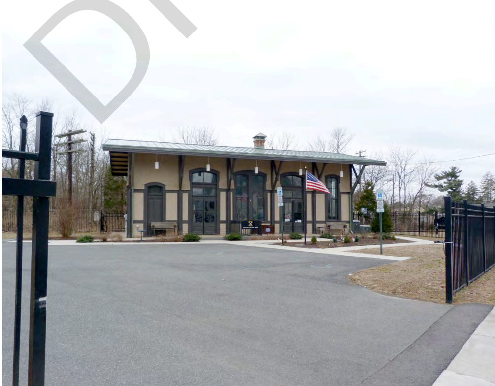
Photograph 0002: View of the site and east elevation, camera facing northwest.
