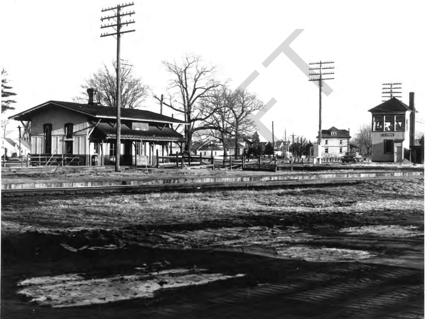
Photograph facing southeast taken in 1963, showing the passenger shelter cut back to just the width of the building and the removal of the north side addition, but the chimney is still intact.
