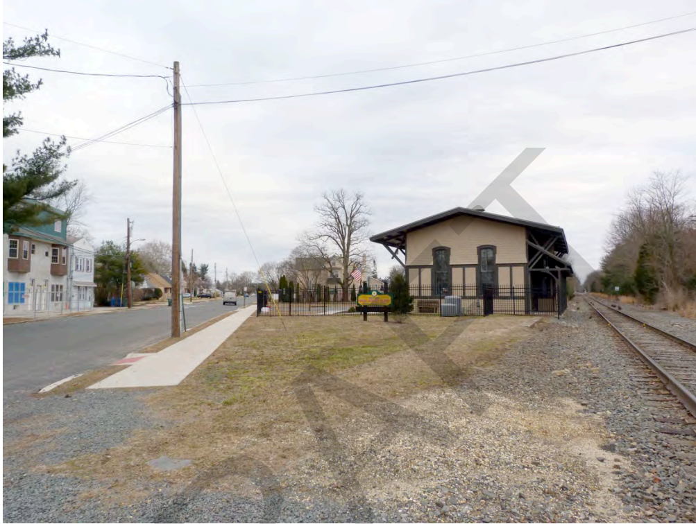
Photograph 0003: View of the site, north elevation, and railroad tracks, camera facing south.
