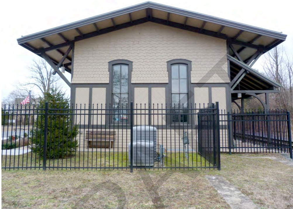
Photograph 0008: View of the north elevation, camera facing south.
