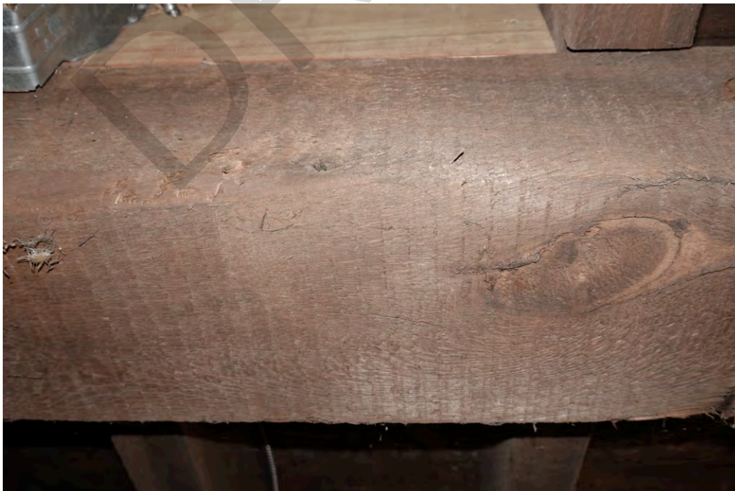
Photograph 0025: Basement framing detail, camera facing east (looking up), showing vertically-sawn lumber.
