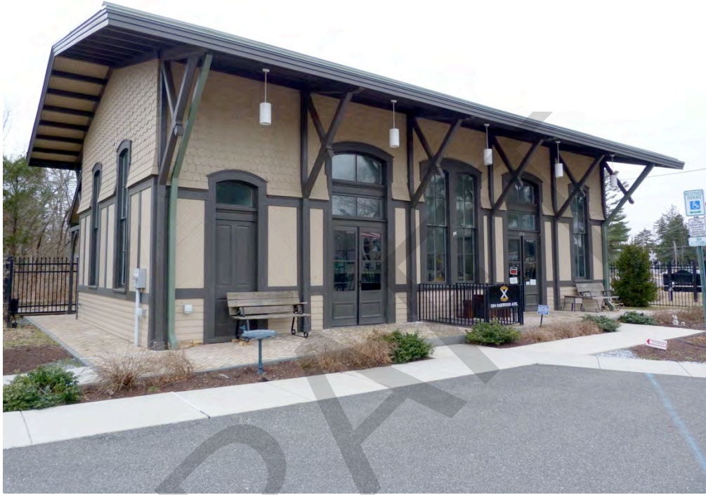
Photograph 0001: View of the south and east (front) elevations of the West Jersey Railroad Glassboro Station, camera facing northwest.
