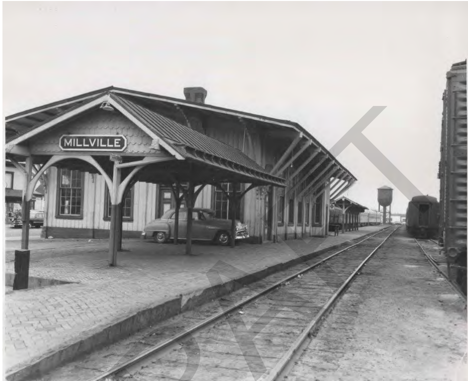
Supplemental Photograph 10: Millville Depot (1867, demolished) MGR/WJRR. This depot was a larger building with eight bays on the eaves elevations. Note the projecting bay near the far end of the elevation, as well as the deep eaves, braces, and board-and-batten siding. The configuration of the interior is not known. (R.L. Long, Photographer, 1956, courtesy of W. George Cook.)
