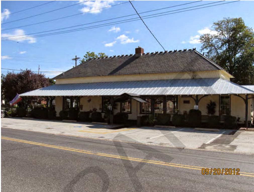
Supplemental Photograph 18: Woodbury Depot (1882), WJRR. This is a Shingle style building with clapboard and shingle siding.
