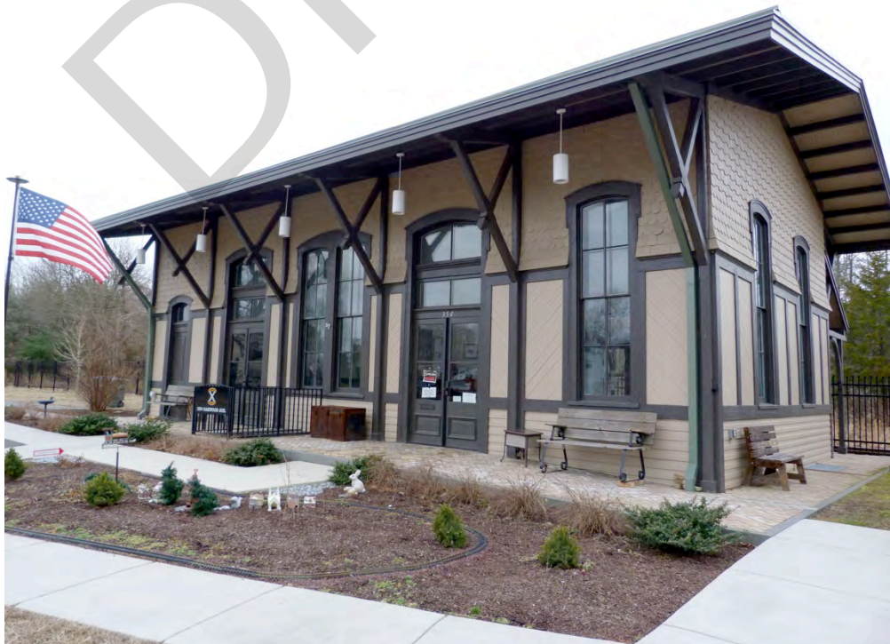
Photograph 0004: View of the east (front) and north elevations, camera facing southwest.
