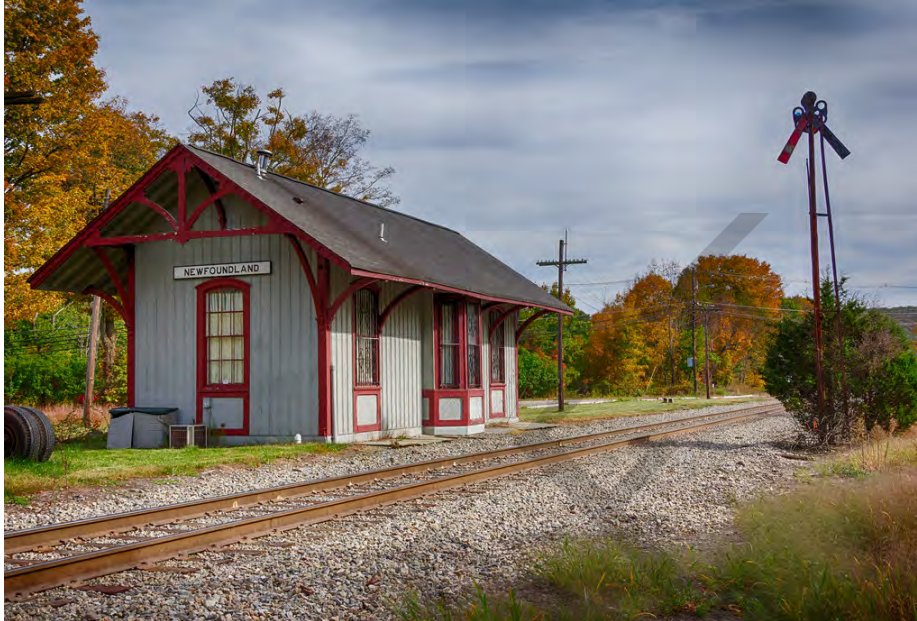
Supplemental Photograph 12: Newfoundland Depot (1872), New Jersey Midland Railway. Note the form, center projecting bay, overhanging eaves with brackets, and board-and-batten siding.
