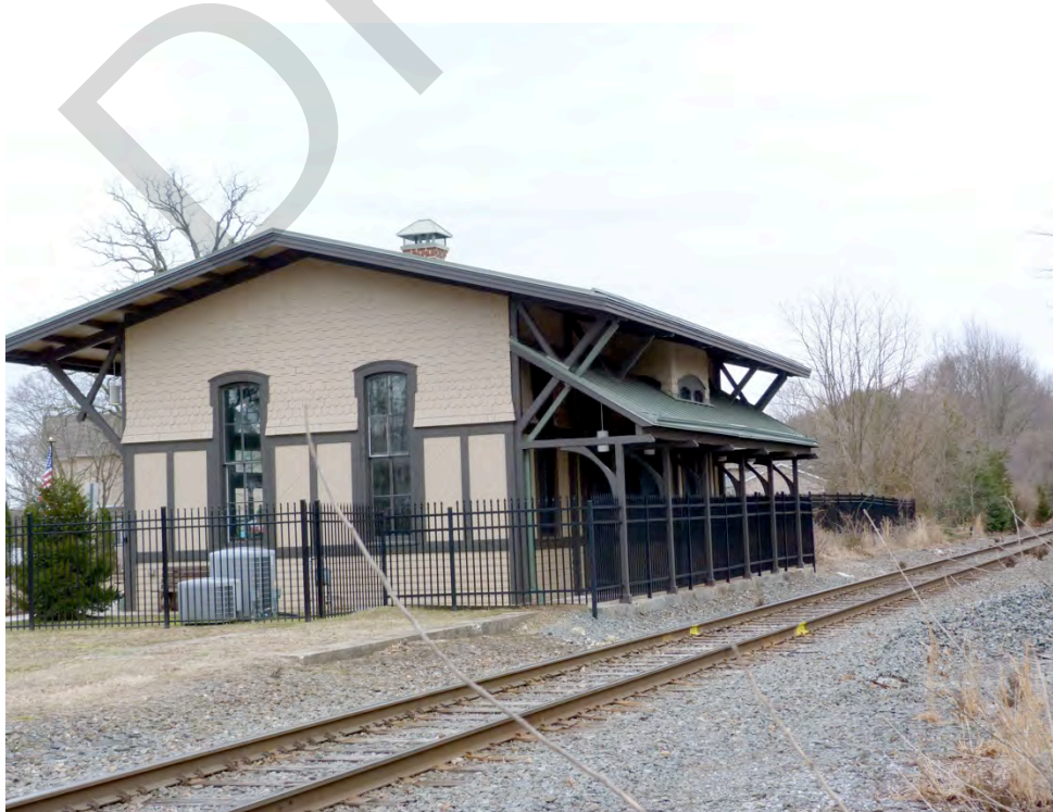
Photograph 0006: View of the north and west elevations and railroad tracks, camera facing southeast.
