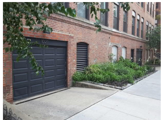
1021 Grand Street (Property ID 158130022), where residential use has been moved above the DFE. Note the recessed infill at the arched openings.
