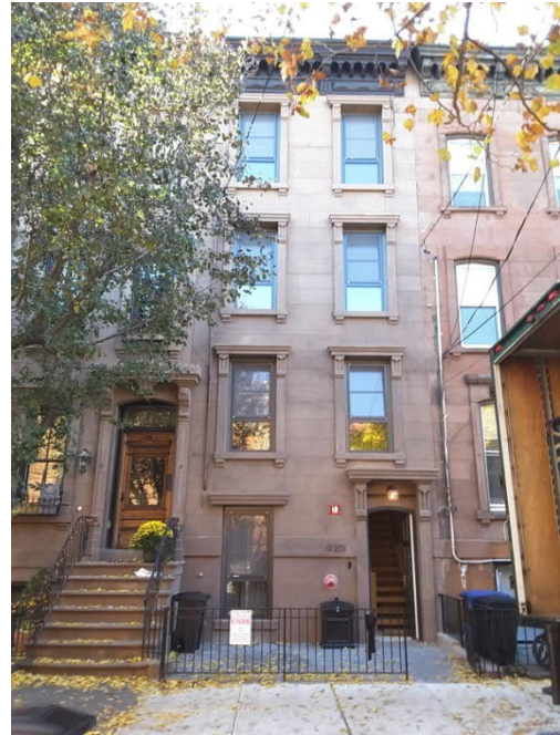
920 Bloomfield Street (Property ID 721301392). Here the basement was eliminated and the floors re-aligned with the first floor above DFE (slightly above sidewalk grade). While this property was still recommended as contributing due to the retained height, massing, upper floor openings, and cornice, its overall integrity is diminished and the streetscape has been adversely affected.
