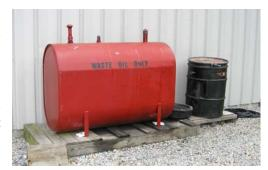
This AST should be on an impervious pad and within secondary containment.
