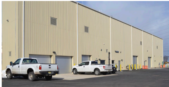
Exterior view of the treatment plant building on Polhemus Lane.
