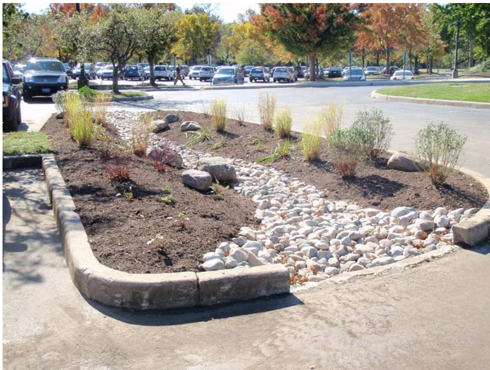
Parking Lot Island Bioinfiltration Cell treats runoff at Subaru Headquarters, Cherry Hill, NJ Camden County Soil Conservation District 319(h) Project Photo by Kathleen Hitchner, October, 2011
