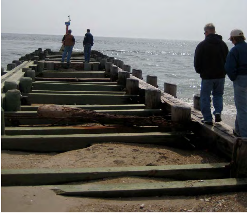
Stormwater outfall pipe, Atlantic Ocean side
