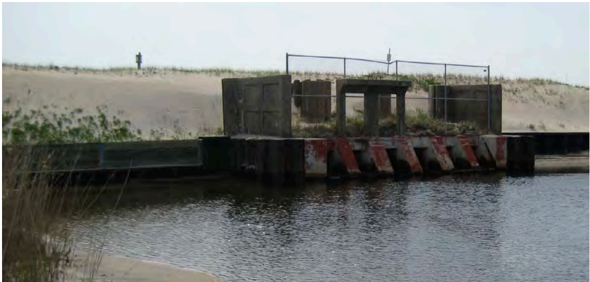
Stormwater outfall, pond side
