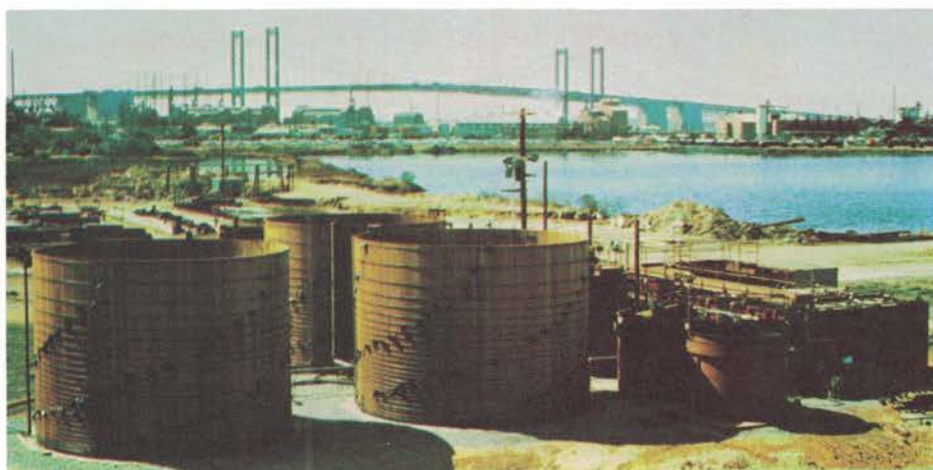
As part of program to bring centralized industrial-municipal wastewater management to the Salem-Gloucester region in South Jersey, this pilot plant was built and operated in 1969-70 at Deepwater under Commission contract. In background are Delaware Memorial Bridges.
