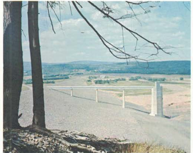
This year marked completion of Beltzville reservoir in the Lehigh Valley, a multi-purpose facility that will be filled by Spring 1971. View is across dam, with water outlet works in foreground.
