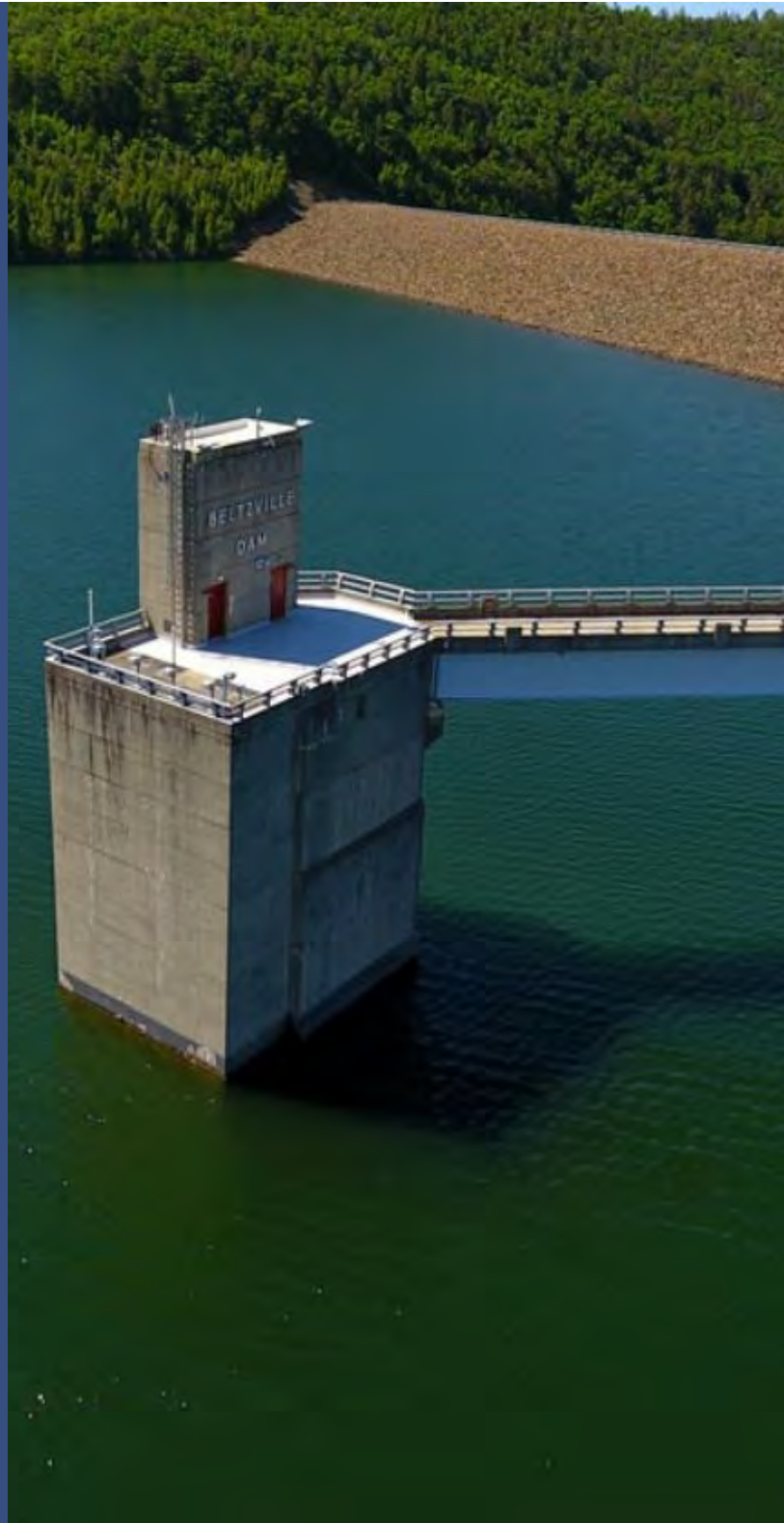
Beltzville Dam was designed and built by the U.S. Army Corps of Engineers (USACE) and completed in 1970. The 13 billion gallon reservoir provides flood damage reduction, water supply, water quality and recreation. Photo Courtesy of USACE, Philadelphia District.
