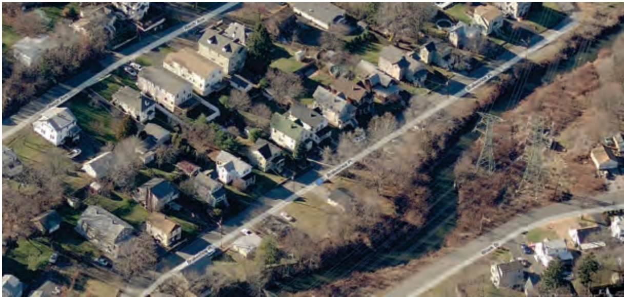
Figure 5: American Foundry Company Worker’s Housing Historic District 25
