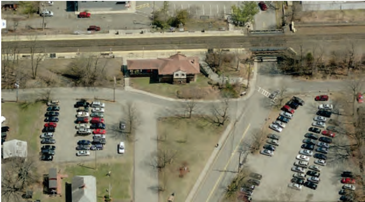
Figure 22: Train station and associated parking lots. 94
