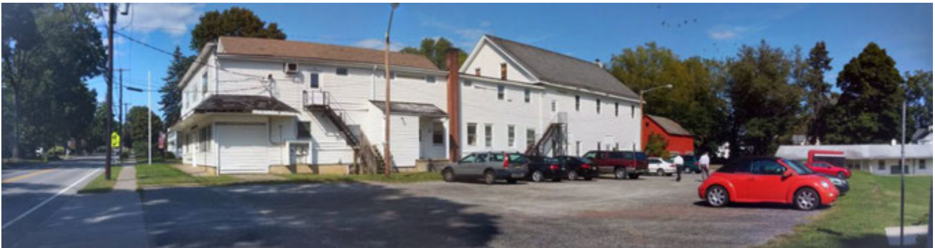
Southerly Side of Building and Lot
