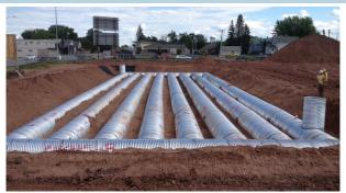
Subsurface Infiltration/ Detention
