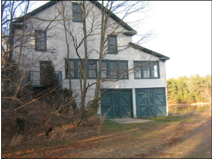
Photo 6: View within Double Trouble State Park toward cranberry packing house adjacent to cranberry bog (12/22/2011).
