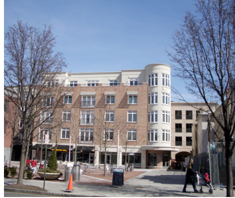
A mixed-use design—Spring Street Garage, Princeton, New Jersey.
