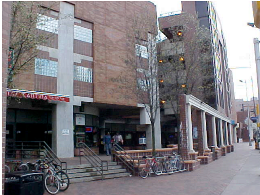
Ferren Deck and Mall, New Brunswick, New Jersey
