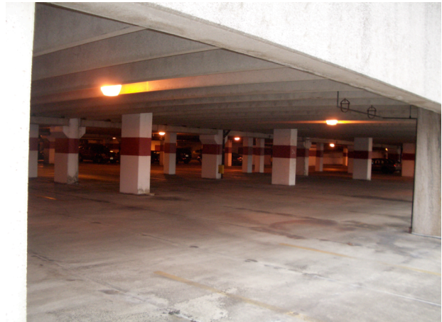
Headquarters Plaza Garage, Interior, Morristown, New Jersey
