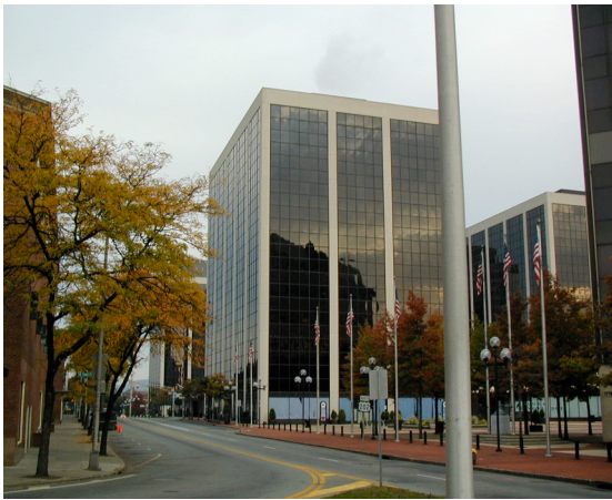
Headquarters Plaza, Exterior, Morristown, New Jersey
