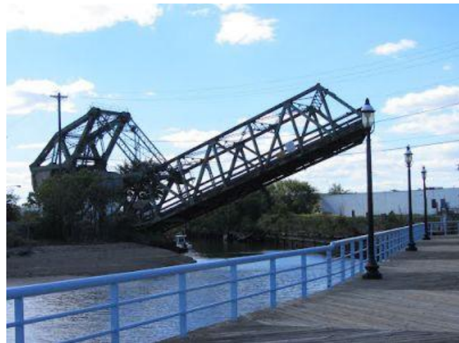
Exhibit 5-11: South Front Street Single-Leaf Bascule Bridge, Union County, New Jersey
