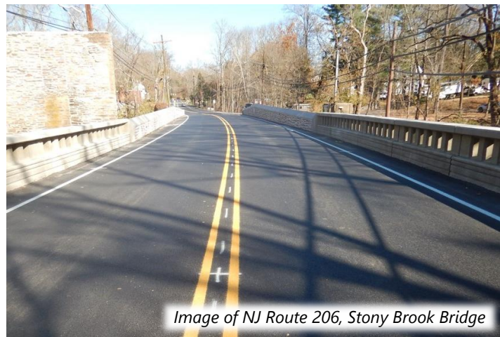
Image of NJ Route 206, Stony Brook Bridge
