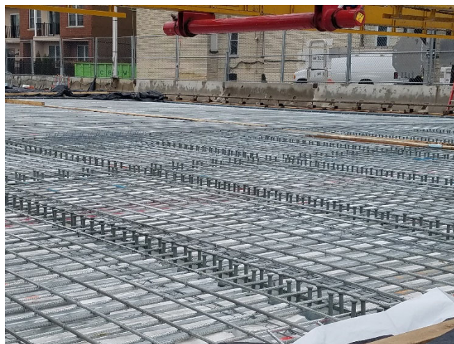
Exhibit 5-16: Galvanized Reinforcing Bars – NJ Route 139
