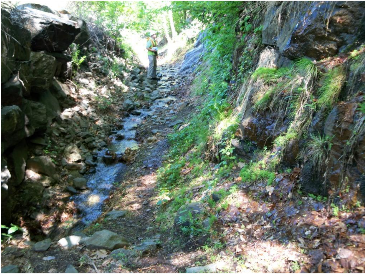
Photo 1 – Existing Drainage Ditch With Stacked Stone Wall to the Left
