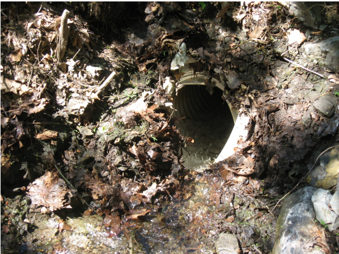
Photo 4 – 18"± Corrugated Metal Pipe Across Route I-80
