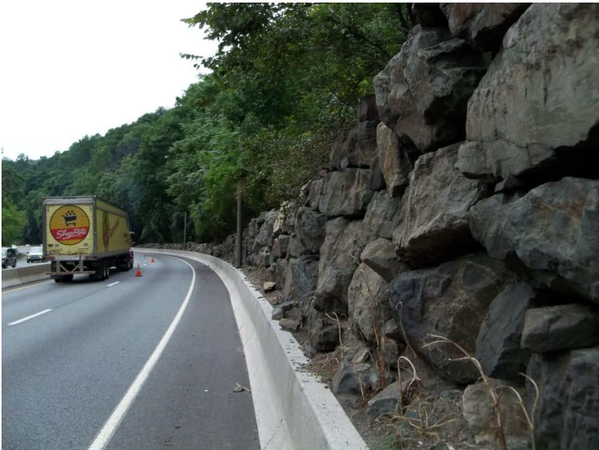
Photo 8 – Close-up View of Stacked Stone Wall on top of Barrier Curb
