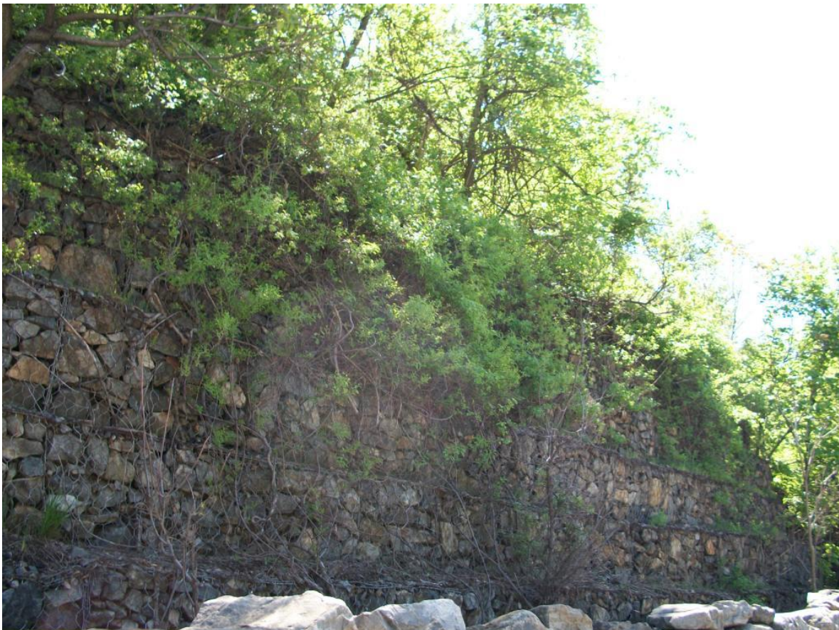
Photo 16 – Existing Gabion Wall
